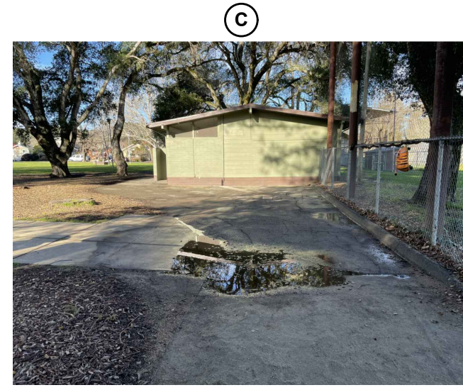
(E) TRANSITION FROM AC TO QUARRY FINES PROTECT QUARRY FINES PATH IN PLACE
