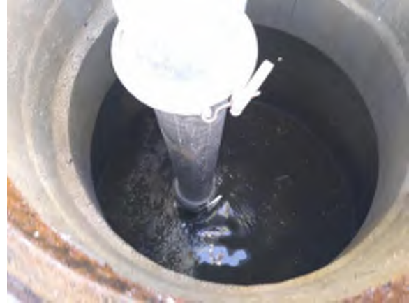
Figure 9: Grit trap at the beginning of cleaning
