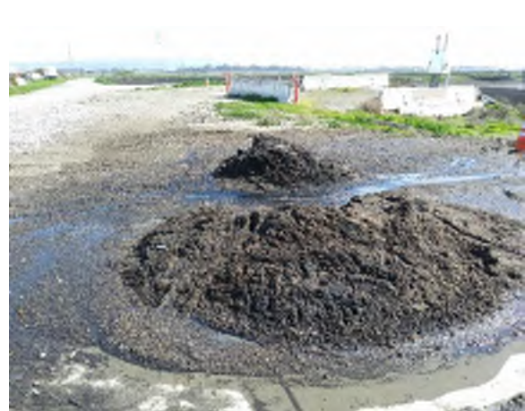
Figure 13: Sediment cleaned from grit trap
