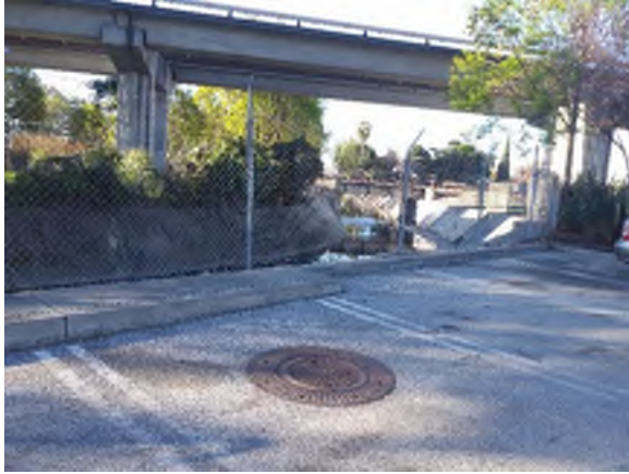
Figure 8: OLSD grit trap location (note the easily accessible location)
