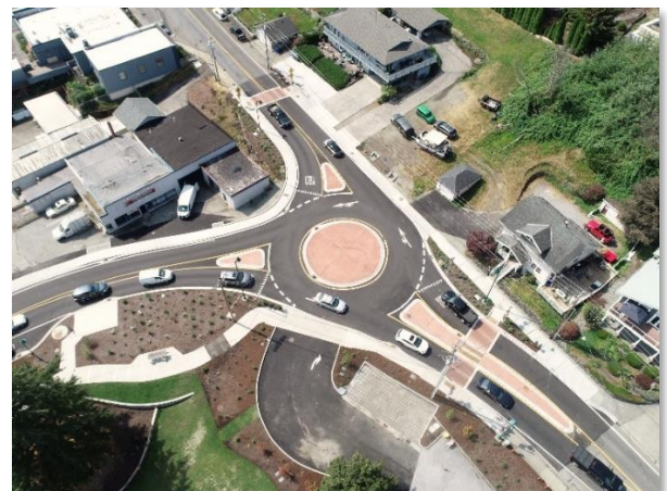
Harborview Dr & Stinson Ave Roundabout, Gig Harbor, WA
