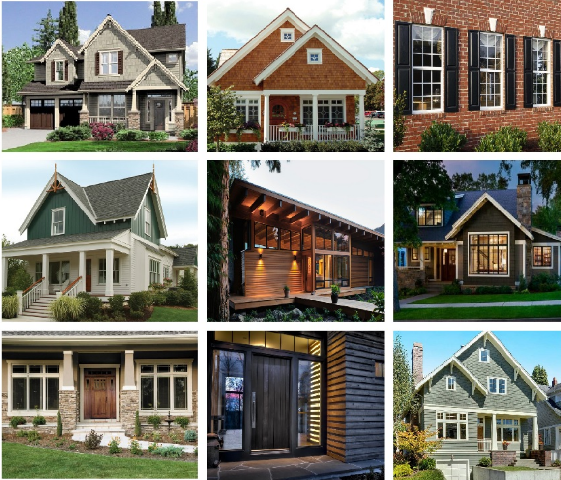
Figure 6. Examples of distinctive window or façade treatments.
