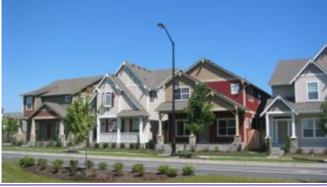
Figure 6. Examples of homes featuring different facade elevations. Notice the different rooflines, entry features, window designs/locations, exterior materials, and colors.
