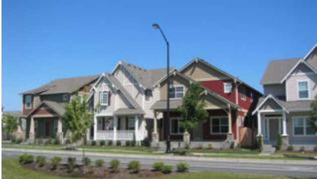
Figure 8. Examples of homes featuring different facade elevations. Notice the different rooflines, entry features, window designs/locations, exterior materials, and colors.
