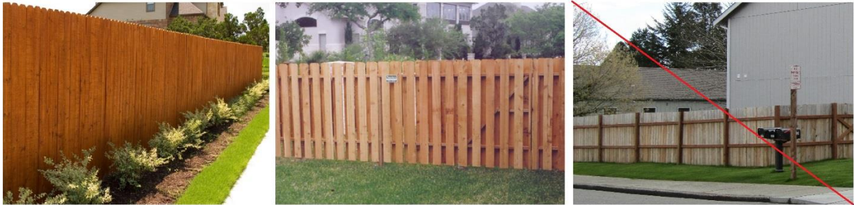
Figure 11: Fence with finished side facing a street (left); Fence finished on both sides (center); Fence with finished side not facing a street (right).
