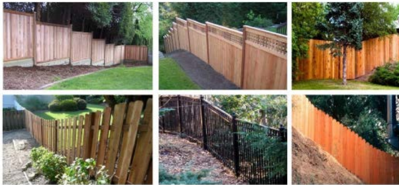
Figure 11: Fences on slopes.
