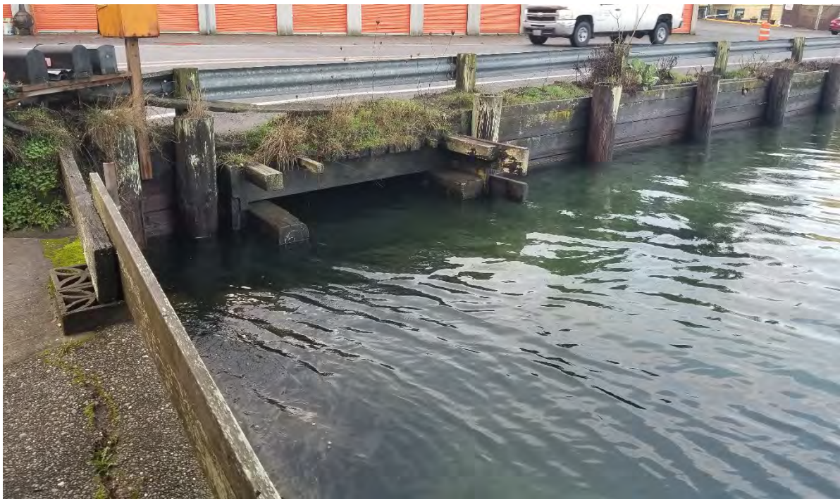
Photo 2-2. Bay Street Culvert at High Tide.
