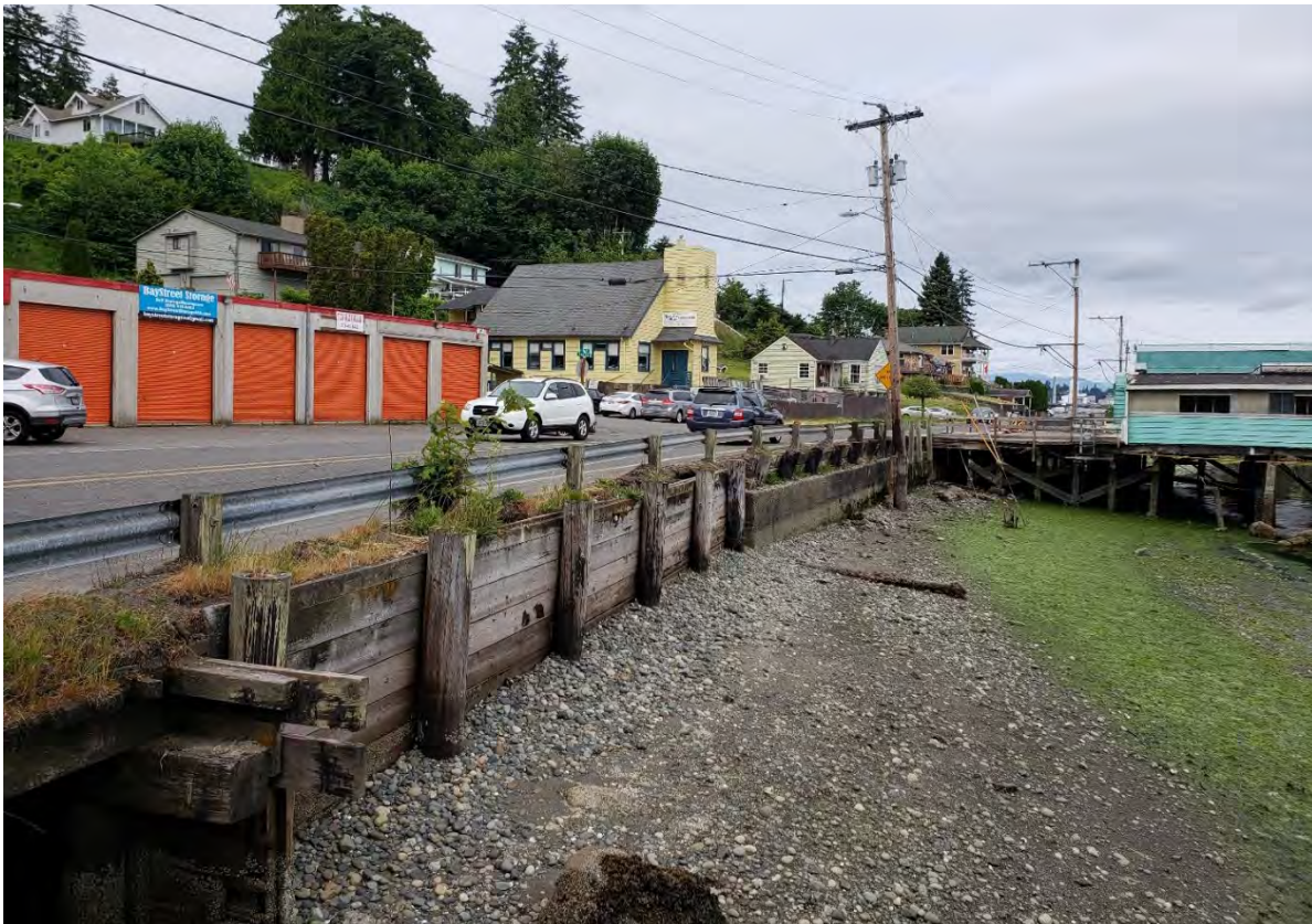
Photo 6-1. Existing Bulkhead at Bay Street.
