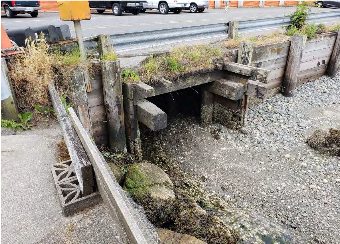
Photo 2-1. Bay Street Culvert at Low Tide.
