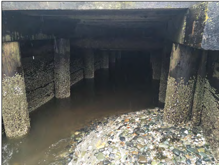
Photograph 4. Inside the Annapolis Creek Bay Street culvert underneath Bay Street.
