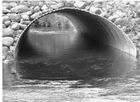
Corrugated Steel Arch Culvert
