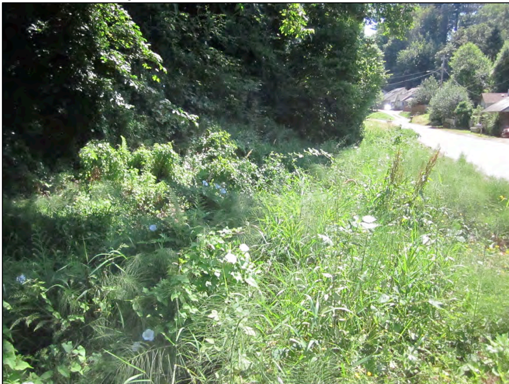
Figure 6. Typical Annapolis Creek channel conditions upstream from Lawrence Street; view is to the south-southwest. View is of a densely vegetated ditch.
