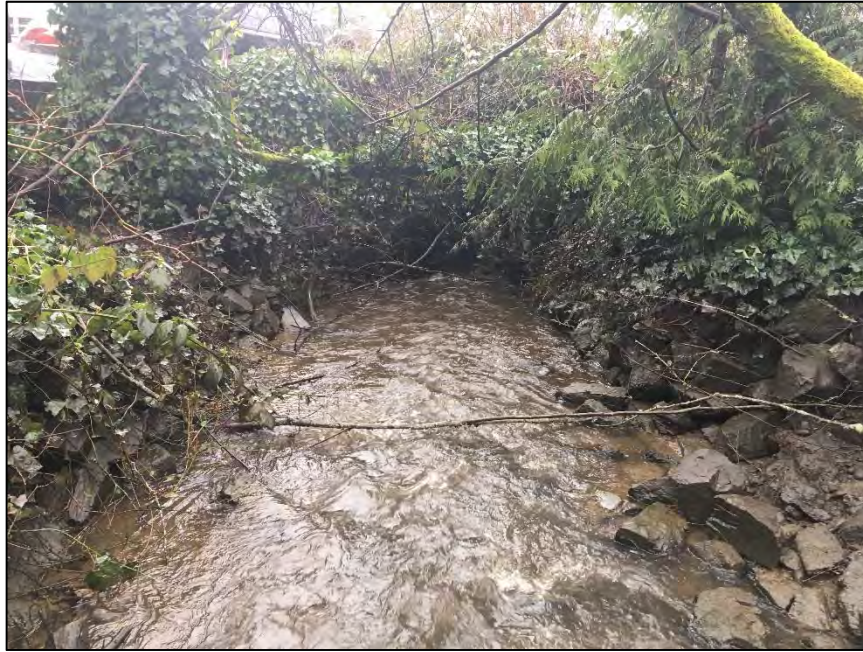
Photograph 5. Annapolis Creek upstream of the Annapolis Creek Bay Street culvert.
