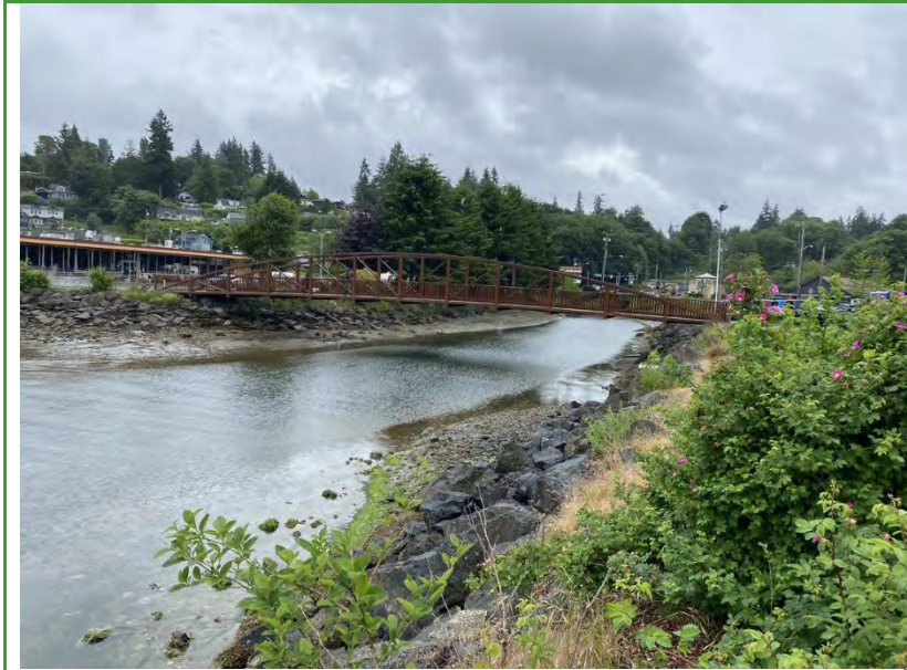
Bridge over confluence of Blackjack Creek with Sinclair Inlet; looking upstream
