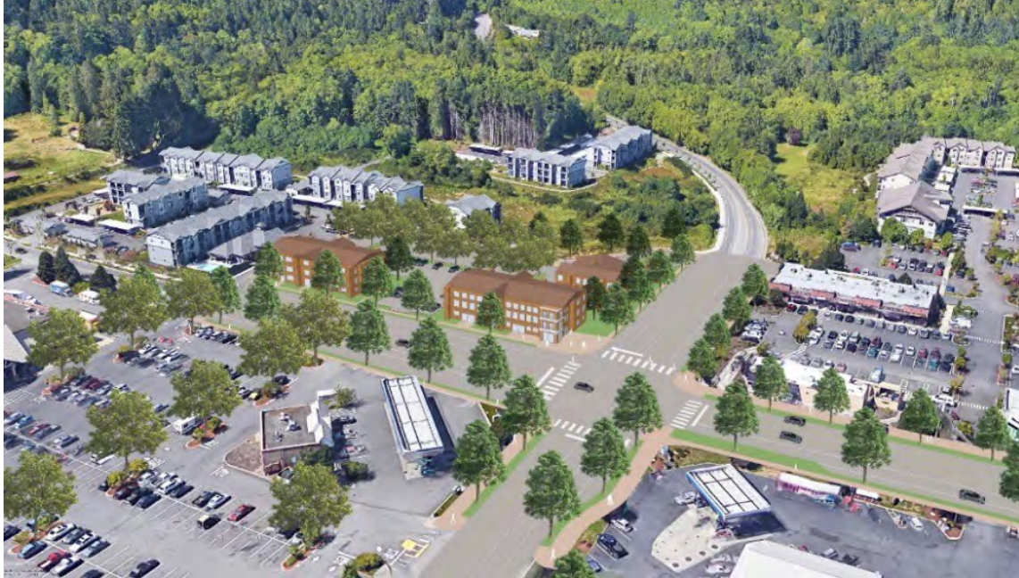
Figure 7: The south end of the Ruby Creek Neighborhood as seen from the northeast, showing the crossroads of Sidney Road SW and SW Sedgwick Road.
