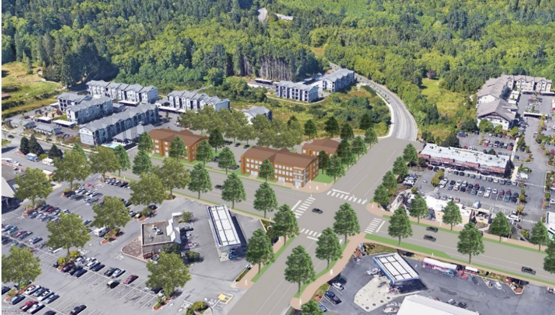
Figure 7: The south end of the Ruby Creek Neighborhood as seen from the northeast, showing the crossroads of Sidney Road SW and SW Sedgwick Road.
