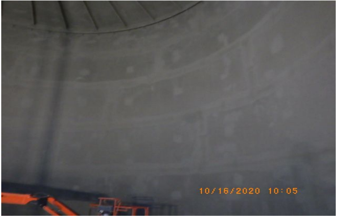
Application of zinc primer to shell
