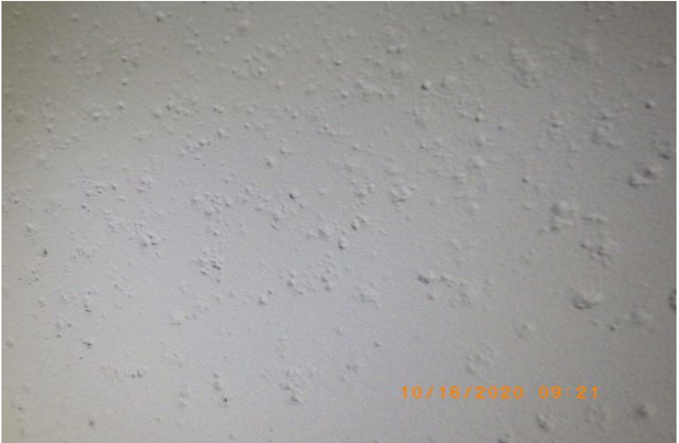
Examples of the pitting found in the webs of rafters – Important to have these areas checked through holiday testing to ensure no pinholes are found
