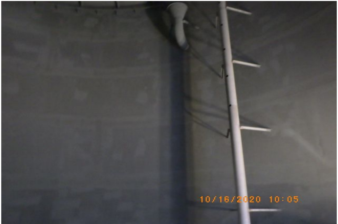
Application of zinc primer to shell
