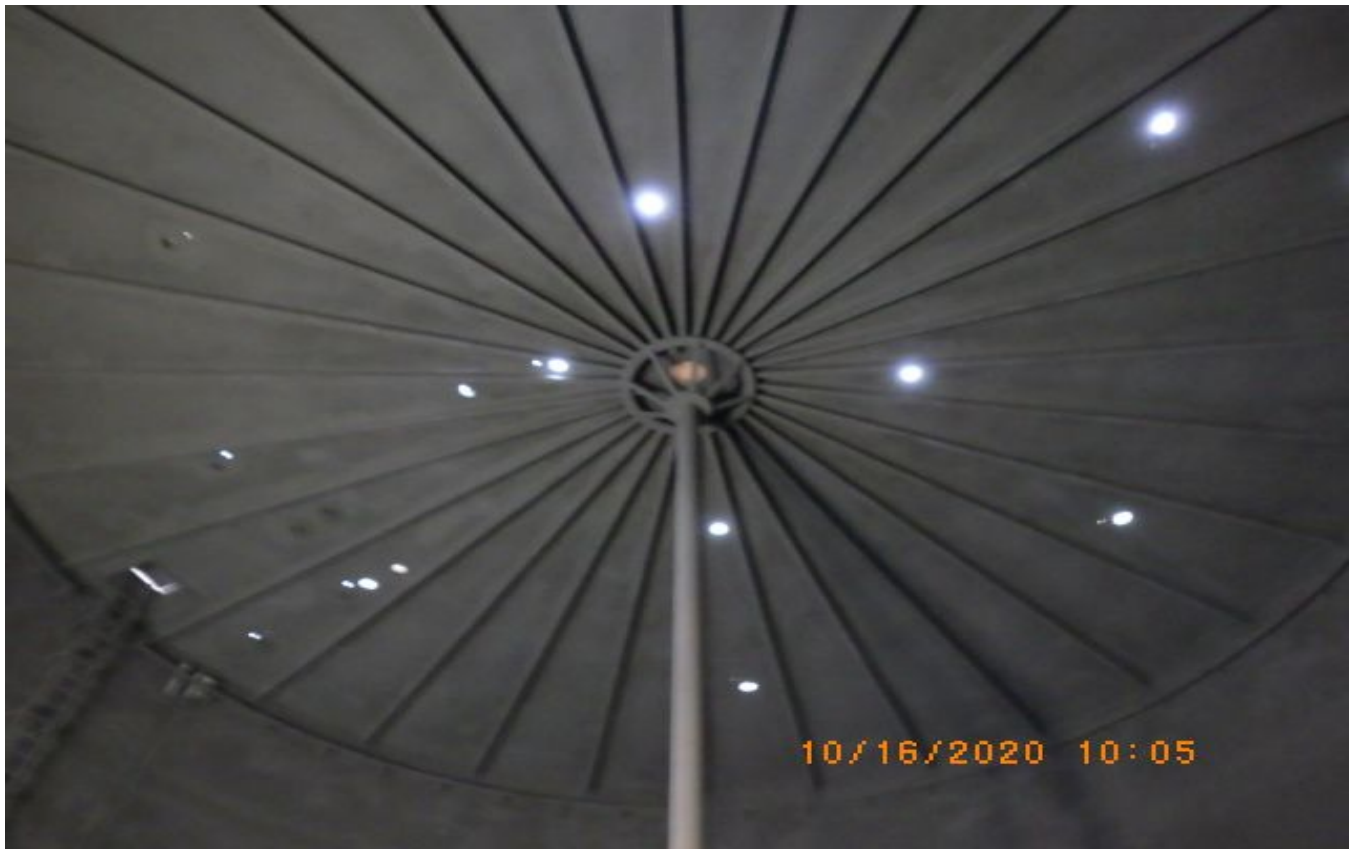
Application of the zinc primer, ceiling and shell
