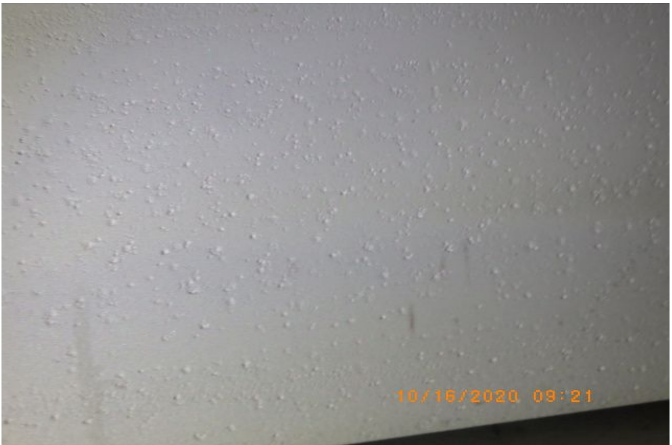
Examples of the pitting found in the webs of rafters – Important to have these areas checked through holiday testing to ensure no pinholes are found
