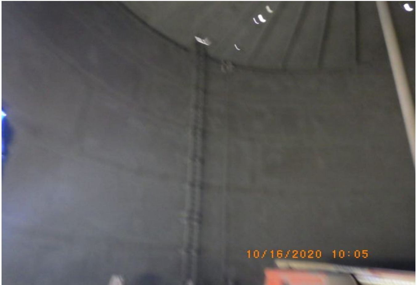
Application of the zinc primer, ceiling and shell
