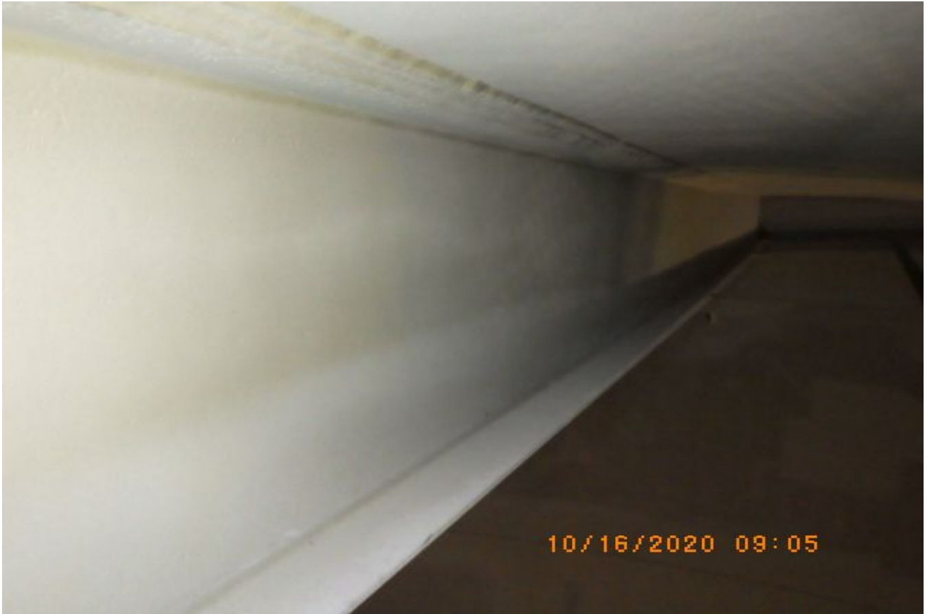
Application of zinc primer in ceiling
