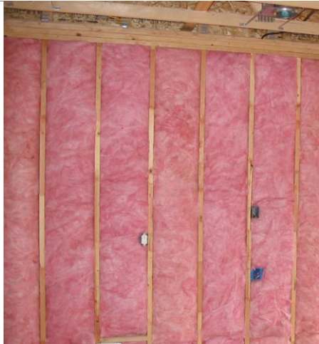
R-21 cavity allowed but not recommended due to potential moisture problems
