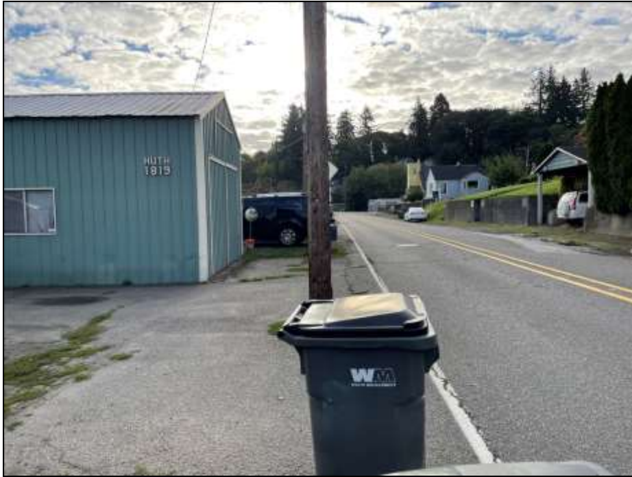
PHOTO ONE: SOUTHEASTERLY VIEW OF BAY STREET, PROPOSED ROAD VACATION AREA TO THE LEFT
