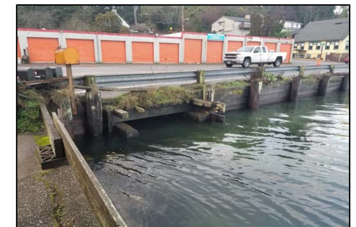
Wood-framed box culvert at high tide
