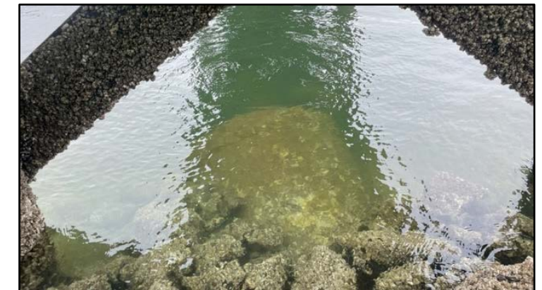
Downstream end of culvert under public dock
