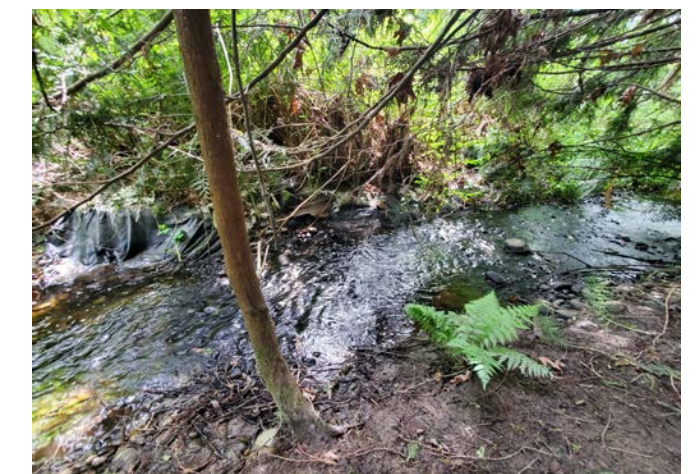
Geotextile fabric-lined upstream right bank
