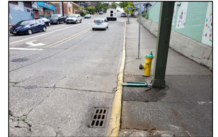
Typical drain inlets in Downtown Basin
