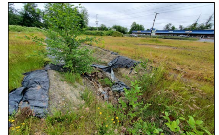
Temporary relief channel dug on northern property
