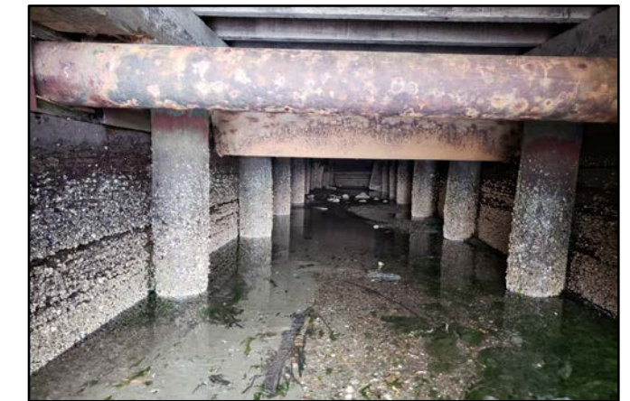
Existing utilities crossing through box culvert
