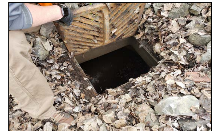
Drainage structure with crossing utility pipes
