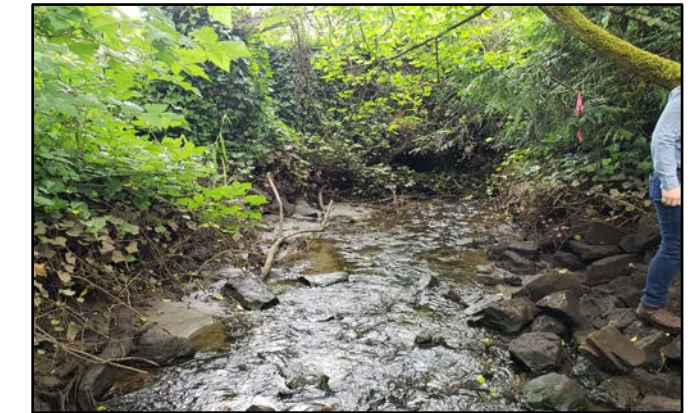
36-inch culvert inlet
