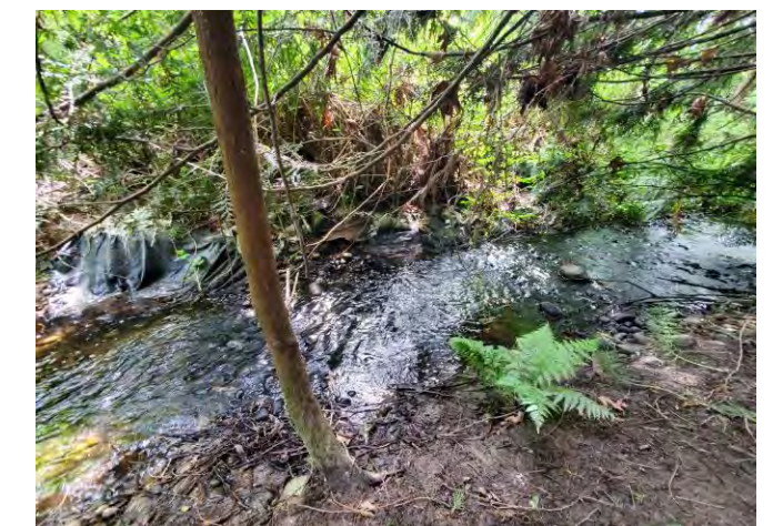
Geotextile fabric-lined upstream right bank
