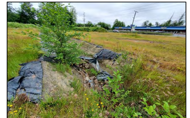
Temporary relief channel dug on northern property
