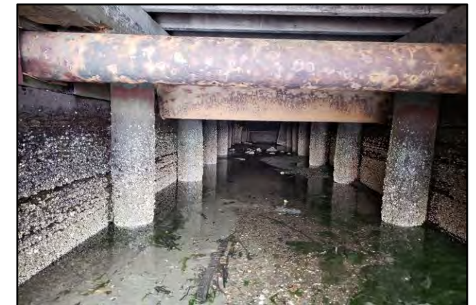
Existing utilities crossing through box culvert
