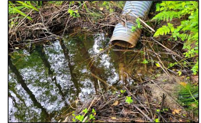
Newly installed stormwater input at the crossing outlet
