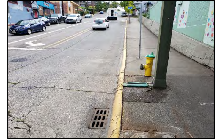
Typical drain inlets in Downtown Basin
