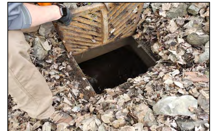
Drainage structure with crossing utility pipes
