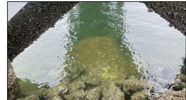
Downstream end of culvert under public dock
