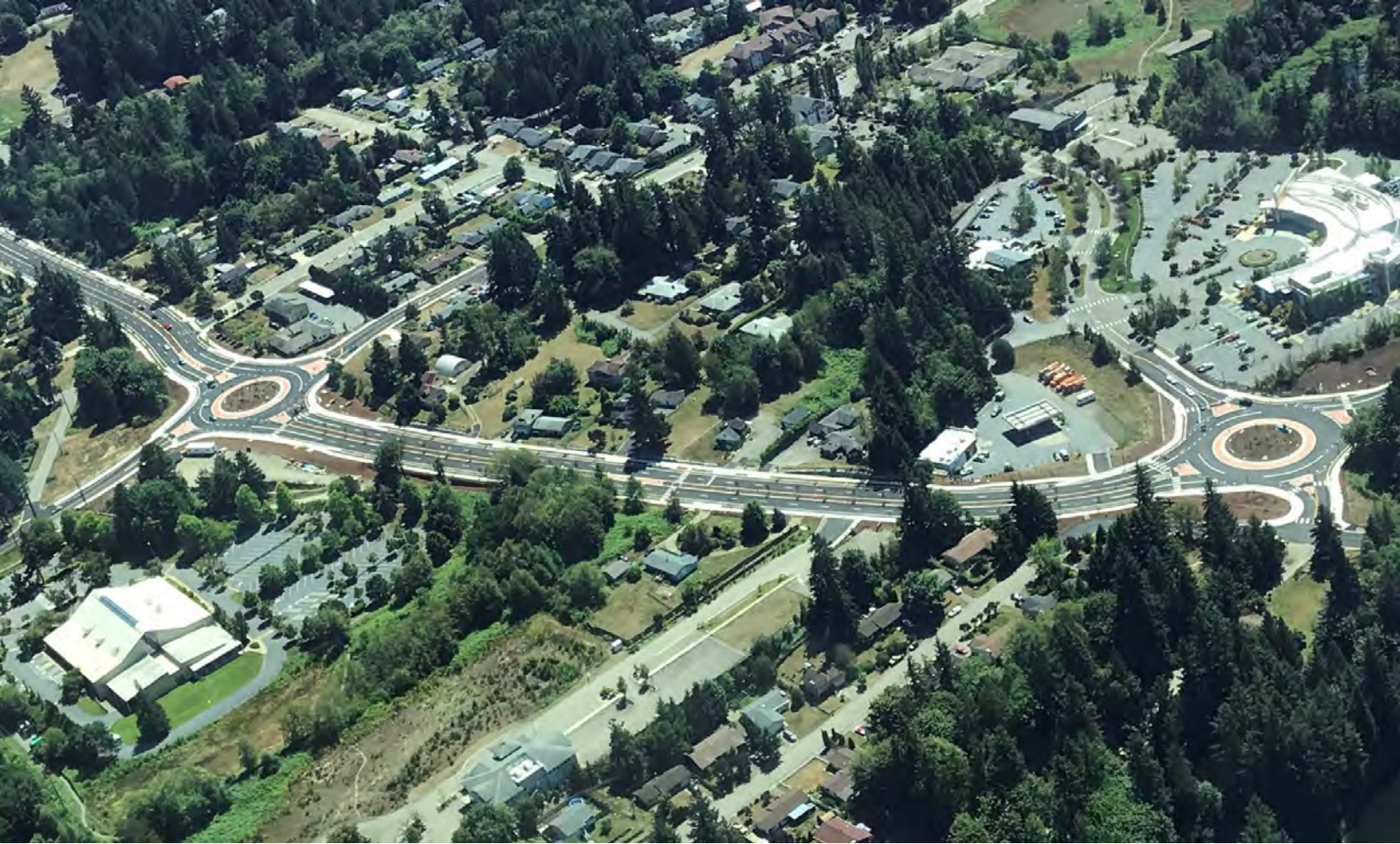
Tremont Street Widening Project, Courtesy City of Port Orchard, Public Works Dept.
