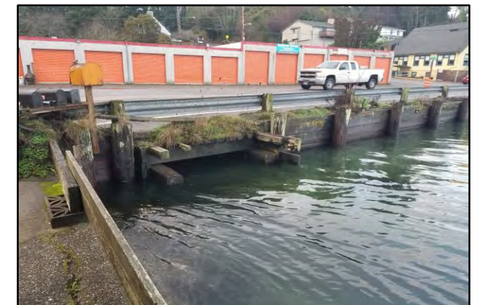
Wood-framed box culvert at high tide
