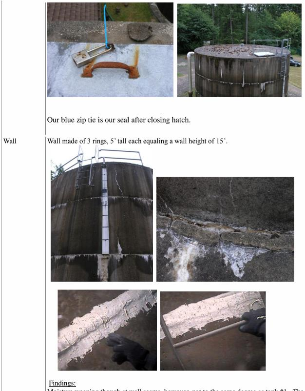
Moisture weeping though at wall seams, however, not to the same degree as tank #1. The inside Aquatapoxy A7 putty application is applied differently and 'neater' than in #1 and may be a significant factor in the quality of the seal.
