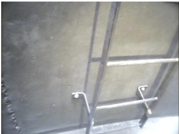
(#15) Interior Ladder Base
