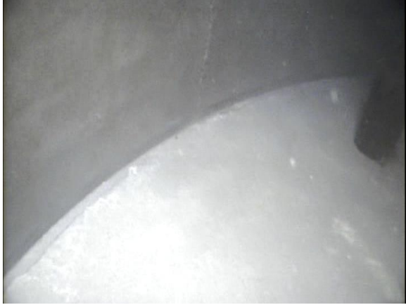
(#19) Floor Wall Seam Quadrant 1
