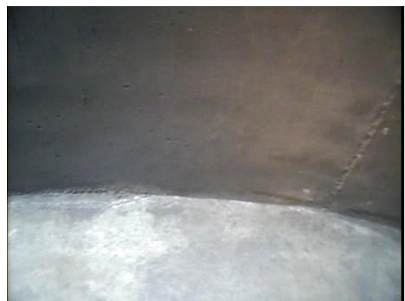
(#24) Floor Wall Seam Quadrant 1
