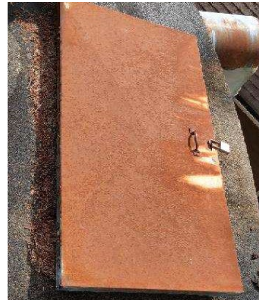
(#11) Roof Access Hatch
