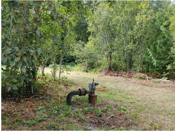
(#1) Site / External Plumbing
