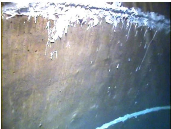
(#21) Wall Course 2 Quadrant 1
