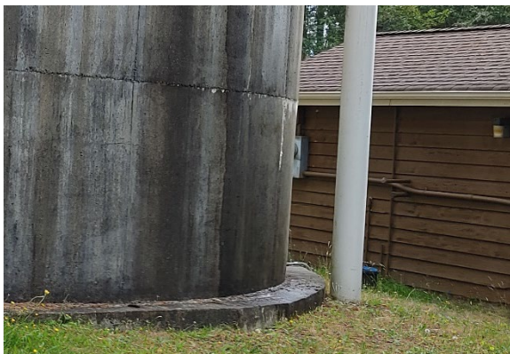
(#2) Foundation / Overflow / Pump house
