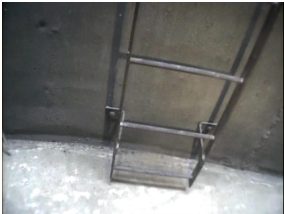
(#20) Interior Ladder Base
