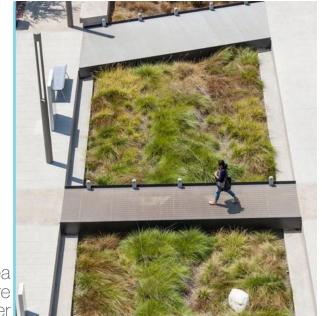
bioretention area to help capture stormwater
