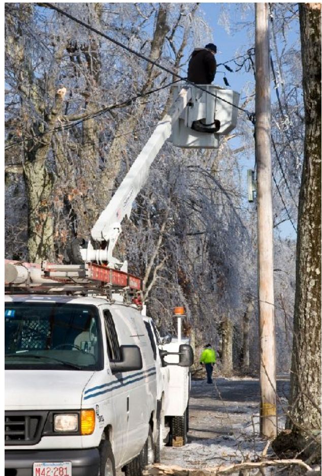
Ice Storm Repair, photo courtesy of CS
