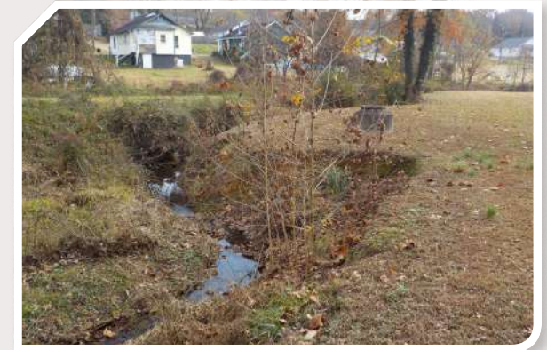
Opportunities for stream bank repair exists along both Cleghorn Creek and the unnamed tributary within park boundaries. Repairing the eroding stream bank can help manage water quality and create safer creek access points. Stream bank repair also opens up potential grant funding from the Clean Water Management Trust Fund (CWMTF).
