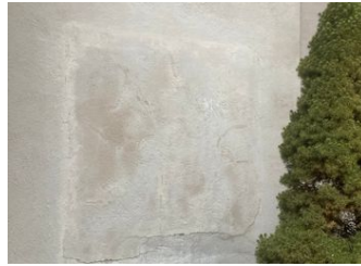
Stucco failing
