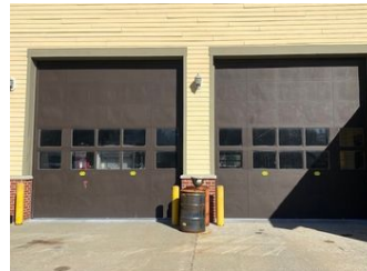
Rear Bay Doors
