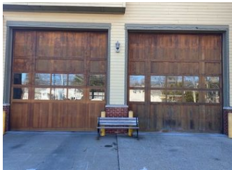
Front Bay Doors
