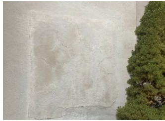
Stucco failing
