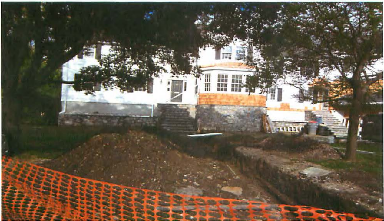
PHOTOGRAPH NO. 8: DAMAGED HOUSE ON MENDOTA AVENUE (INDIAN VILLAGE) MAY 1, 2012
