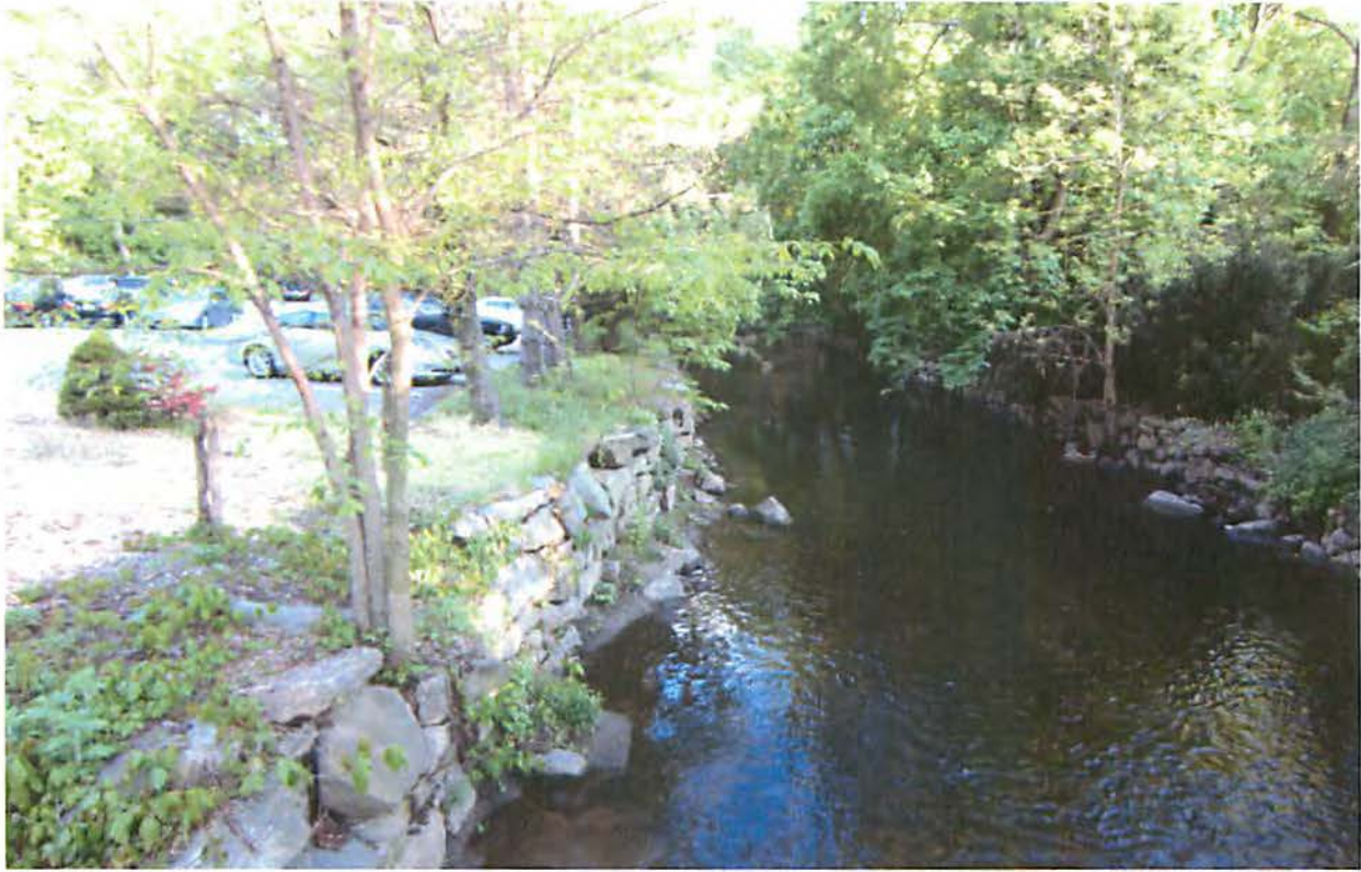
PHOTOGRAPH NO. 9: BLIND BROOK DIRECTLY DOWNSSTREAM OF THE HIGHLAND ROAD BRIDGE - MAY 1, 2012
