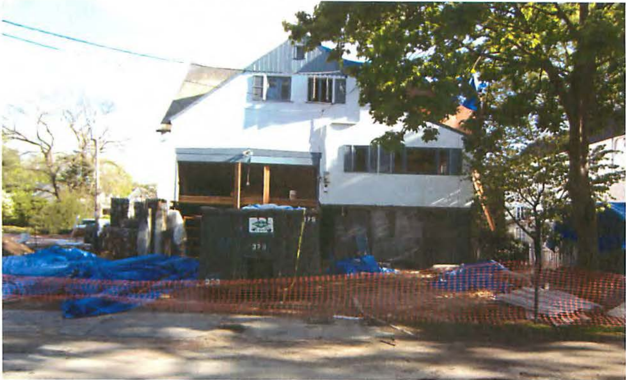
PHOTOGRAPH NO. 7: DAMAGED HOUSE ON MOHAWK STREET (INDIAN VILLAGE)MAY 1, 2012
