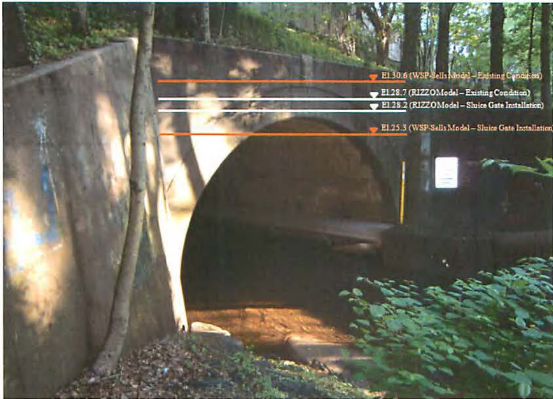
Figure 3: Representation of hydraulic conditions at the I-95 Culvert for the 50-year flood
