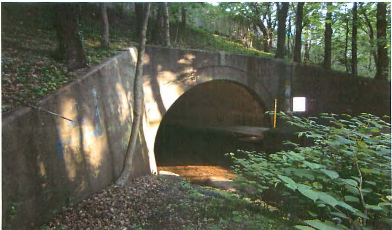
PHOTOGRAPH NO. 10: NEW ENGLAND THRUWAY CULVERT (I95) - MAY 1, 2012
