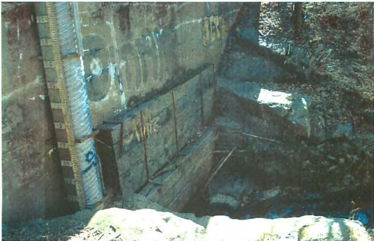
PHOTOGRAPH NO.2: BOWMAN AVENUE DAM - OUTLET OPENING WITH TIMBER LOGS - FEBRUARY 13, 2012
