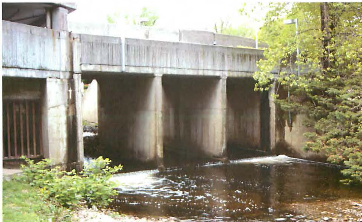
PHOTOGRAPH NO. 4: RIVERVIEW AT PURCHASE CULVERT - MAY 1, 2012
