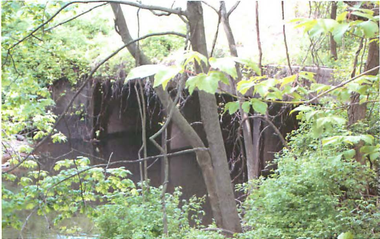
PHOTOGRAPH NO. 5: CROSS WESTCHESTER EXPRESSWAY (I-287) CULVERT MAY 1, 2012
