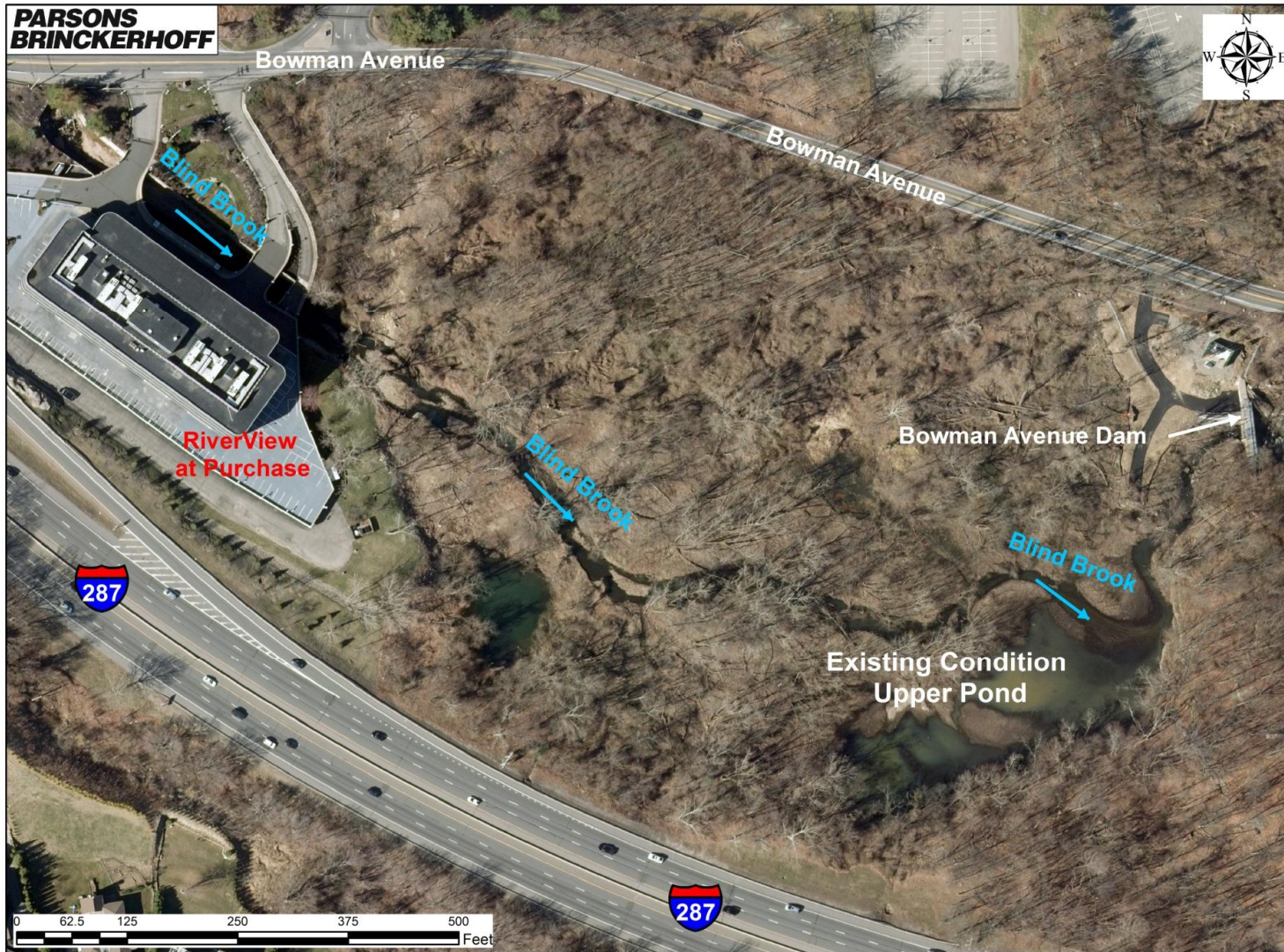
Figure 34 - Aerial Image of Existing Condition Upper Pond
