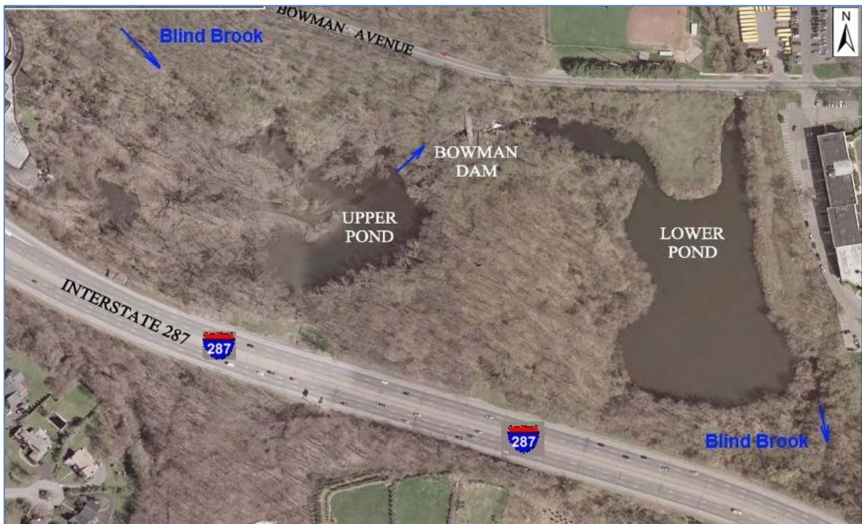
Figure 21 - Existing Condition Aerial Image of Bowman Avenue Dam and Upper Pond and Lower Pond (Scale 1:200')
