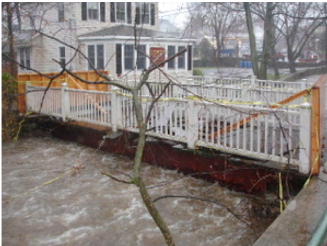
Flooded bridge over Blind Brook (Sara Goddard)
