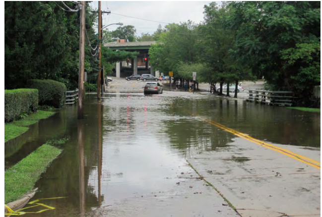
Severe flooding on Highland Avenue during Hurricane Irene (Alexander Breinin)
