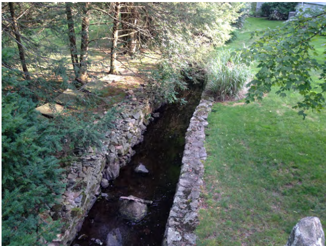
Blind Brook mostly flows through a channel as it passes through Rye.
