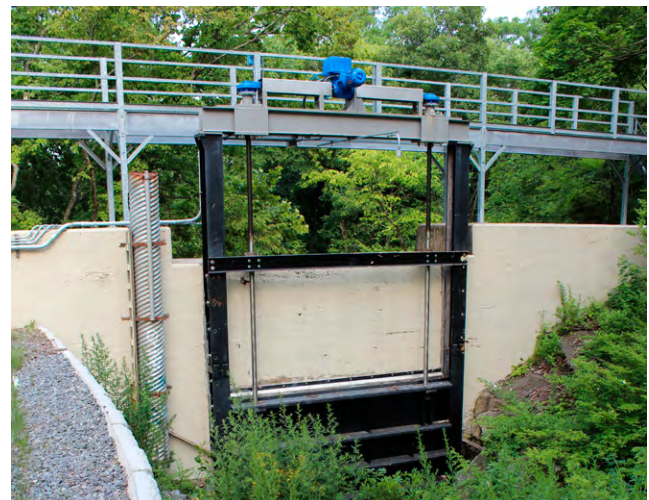
Sluice Gate at the Bowman Avenue Dam.
