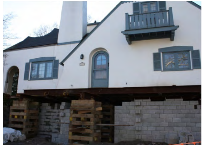
House elevation in progress (Holly Kennedy)
