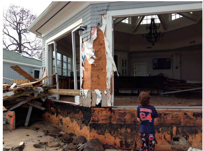
Damage at the Shenorock Shore Club following Hurricane Sandy (Sara Goddard)
