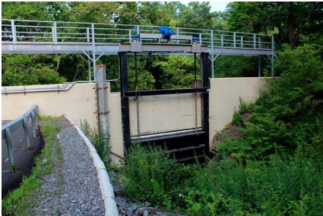
The sluice gate at the Bowman Avenue Dam
