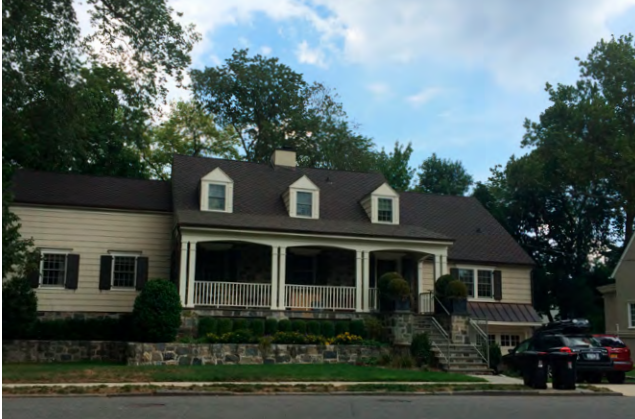
Many homes within the floodplain have been elevated, at great cost to the homeowners.
