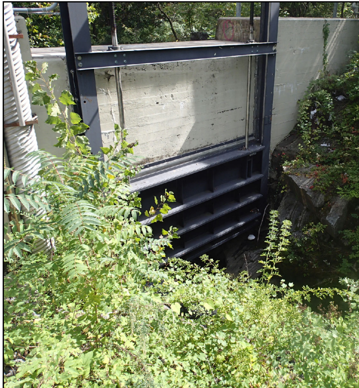
Sluice Gate Photograph - 9/21/2016
