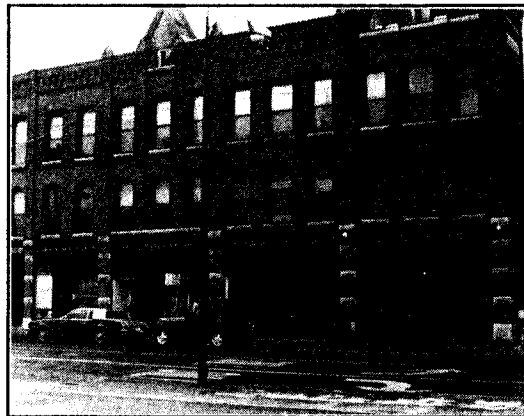
Signs should be coordinated in height and proportion with those on neighboring buildings
