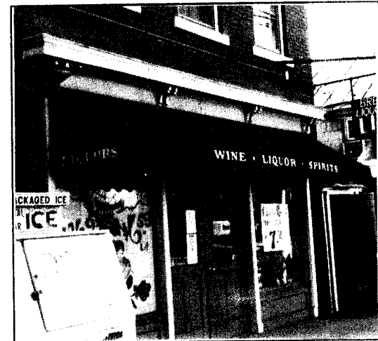
Bottom: Words should be printed on the valence of the awning. Awning does not interfere with architectural detail.
