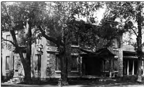
Sackets Harbor Bank Building Before
