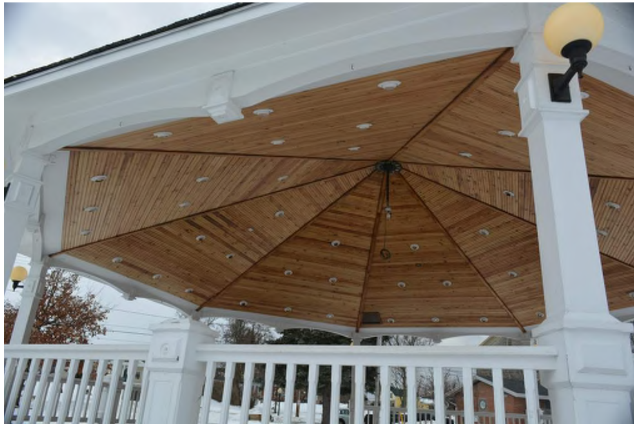
11 EXISTING BEADBOARD CEILING SCALE: 12" = 1'-0"
