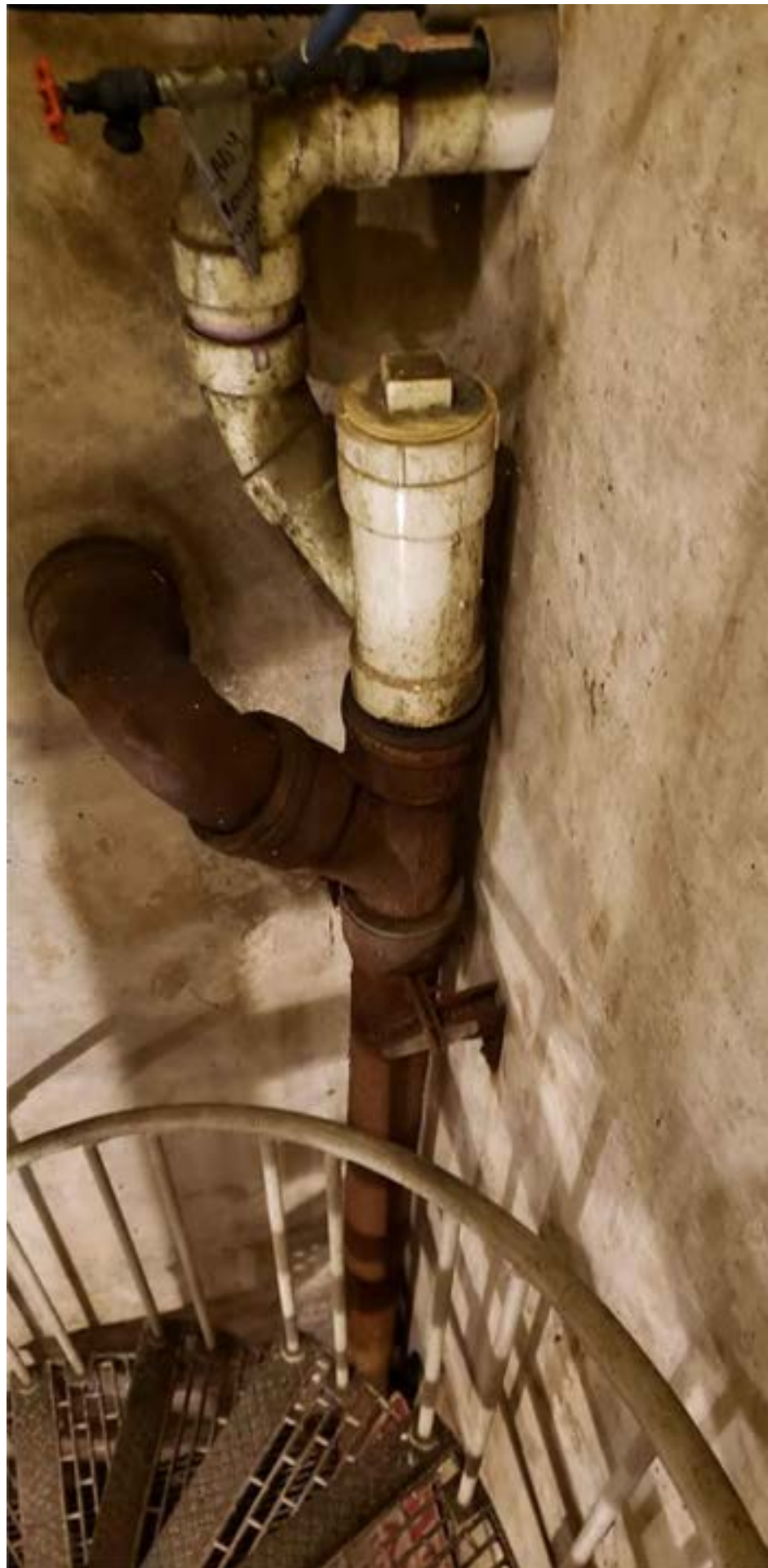
EXISTING INTERIOR SANITARY PIPE FOR FORCE MAIN CONNECTION
