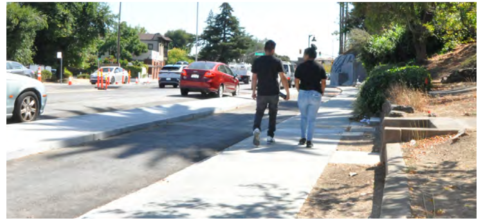
Improvements along 2nd Street, part of the 3rd Street Improvement Project, aim to improve multimodal safety while reducing vehicular congestion.
