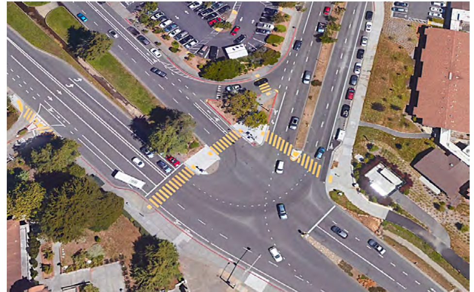
Miller Avenue and Camino Alto intersection.
