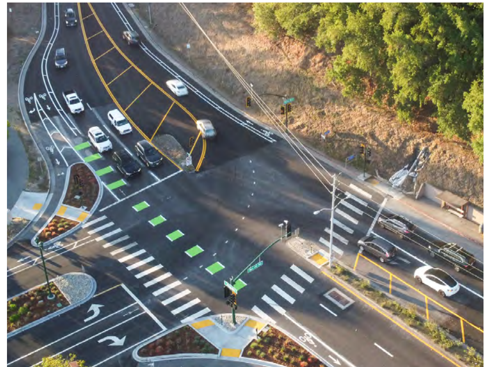
Recent improvements at the intersection of Magnolia Avenue and Bon Air Road included a bicycle lane and traffic calming.
