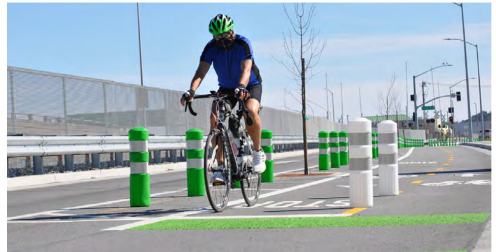
Recent improvements on Francisco Boulevard West increase safety and comfort for cyclists.
