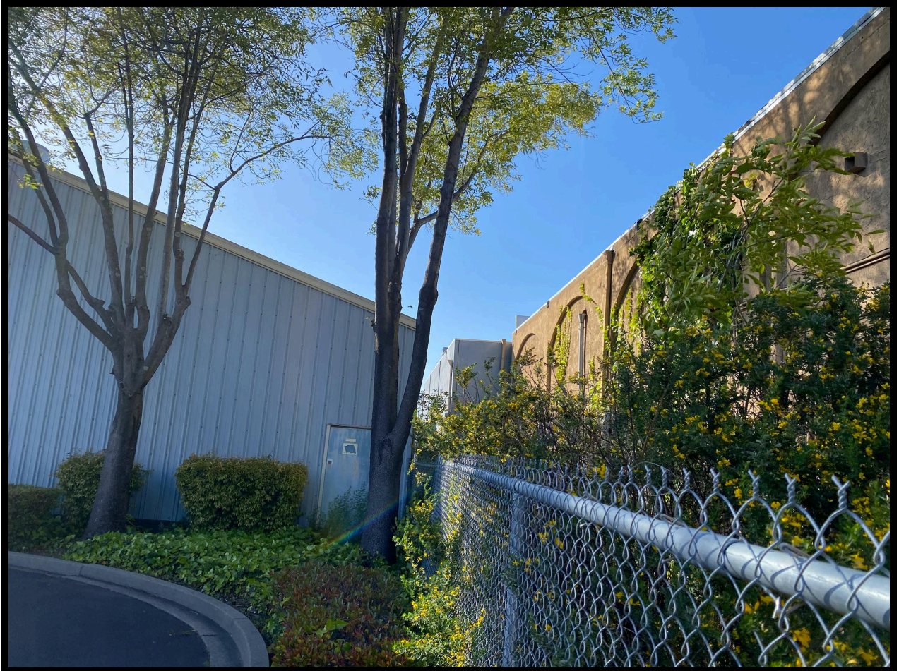
This shows the gap between the Northeast side of the building(left) and the next building over(right). 25 Dodie runs right up to the property line on this side.
