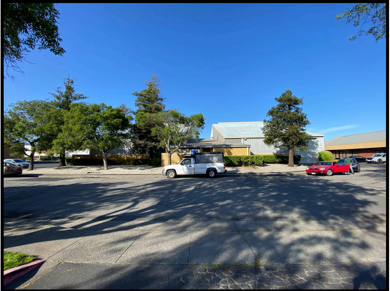
Wide angle shot of the Southwest facing side. This side also faces Dodie street and there is no adjacent building on this side.
