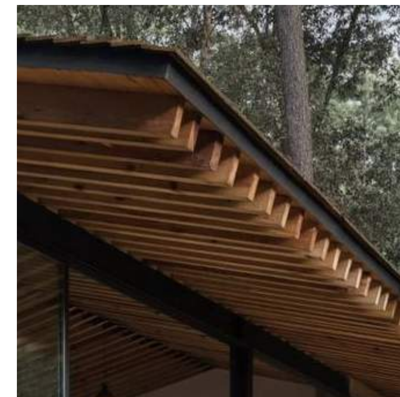
10 ENGINEERED WOOD RAFTERS
