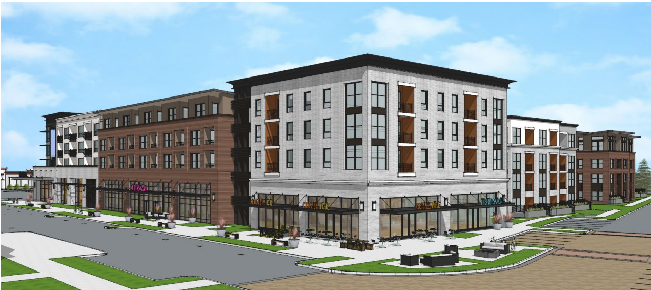
View A: Southwest Corner of Residential 5 facing the Townsquare (Before)
