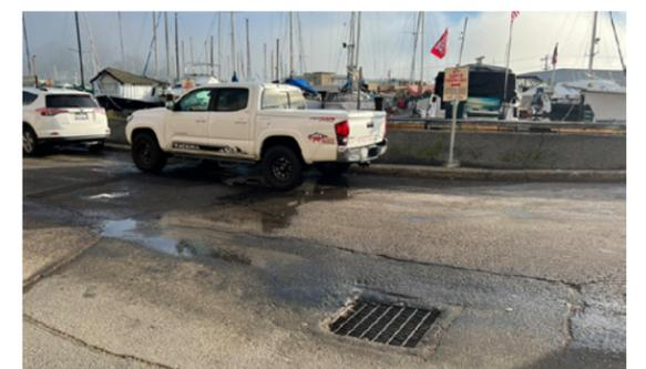
Development on top of former marsh is unstable, causing paved surfaces to crack.
