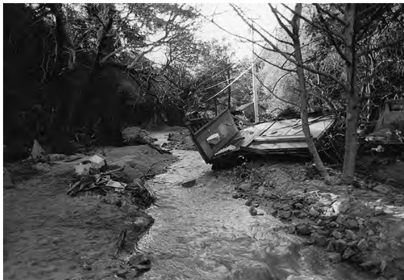
Figure 3.107: Damage in Inverness from 1982 Storm
