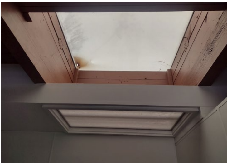
Figure 25. Skylights in the locker room, notice the two different layers and materials (GA, 2025)
