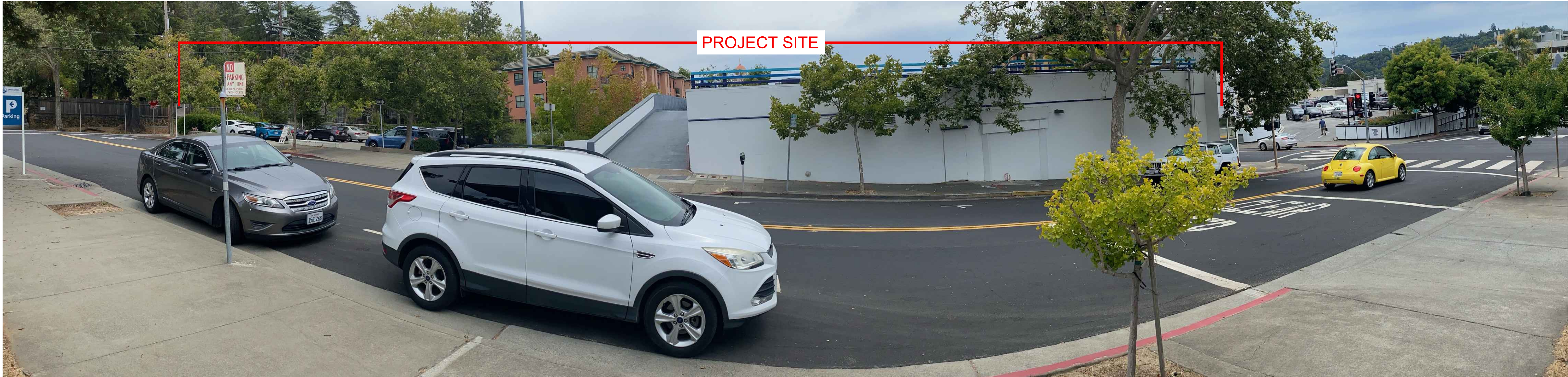
1. VIEW FROM C STREET - FACING EAST
