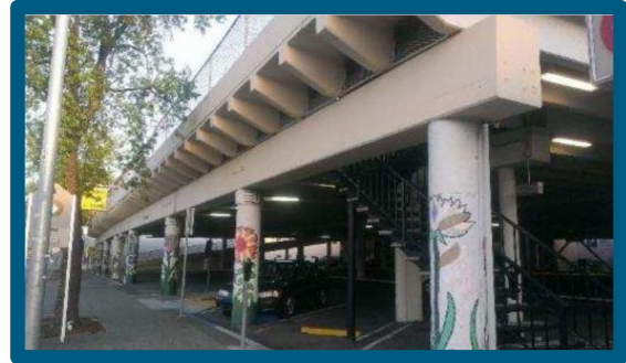
3 rd and Lootens parking structure
