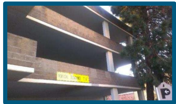
3 rd and A parking structure
