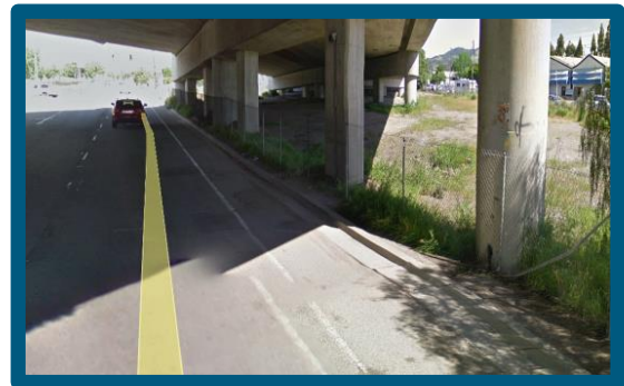
Bellam Blvd under the Highway 101 overpass
