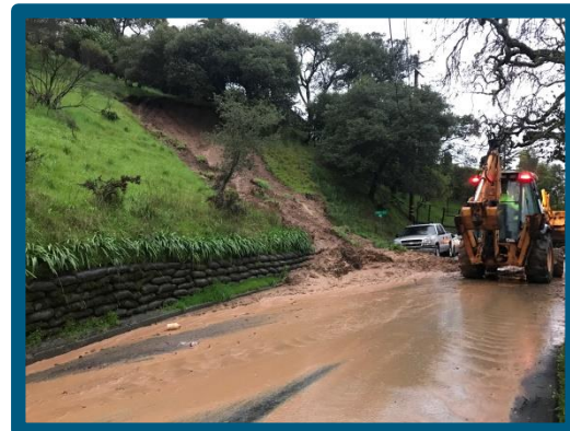
Emergency work performed for slide repair
