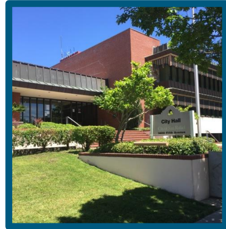
Landscaping outside of City Hall entrance
