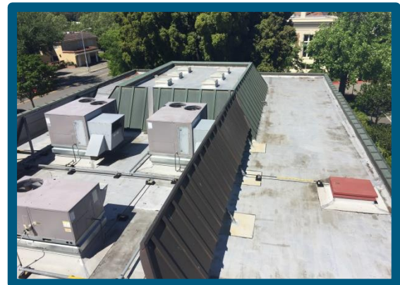
City Hall roof from above
