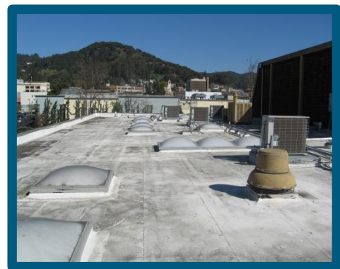
B Street Community Center Roof
