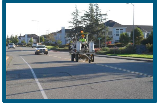
Public Works streets staff operating the road striper
