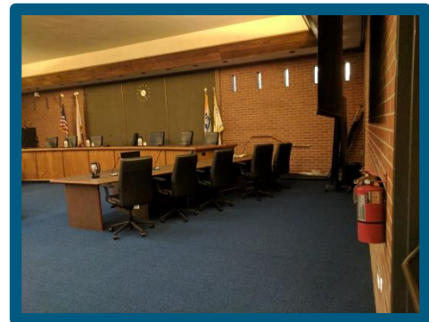
Fire extinguisher in the City Hall Council Chambers
