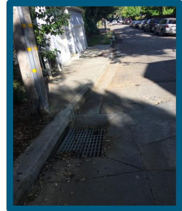
Curb and gutter at East and Jessup
