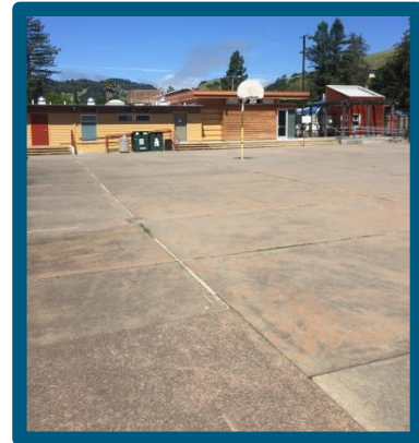
Basketball court at TL Community Center
