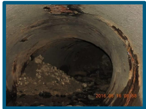
Corrugated metal pipe underneath Larkspur Street
