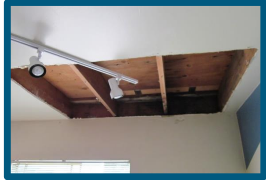
Example of emergency roofing work at Fire Station 57
