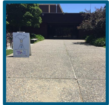
Concrete patio, facing front entrance
