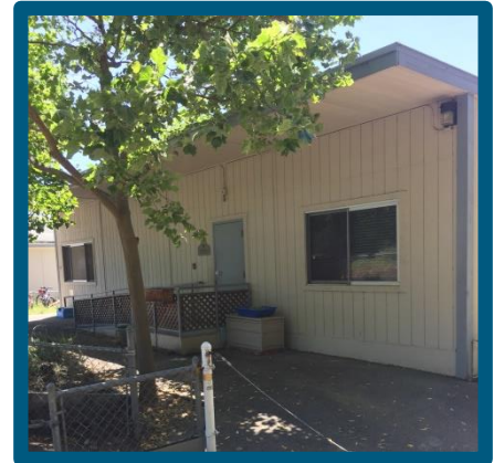
Portable building to be replaced at Dixie
