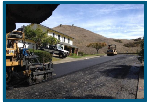
Street resurfacing work
