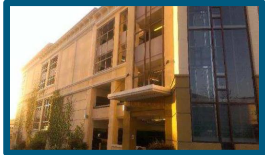
3 rd and C parking structure
