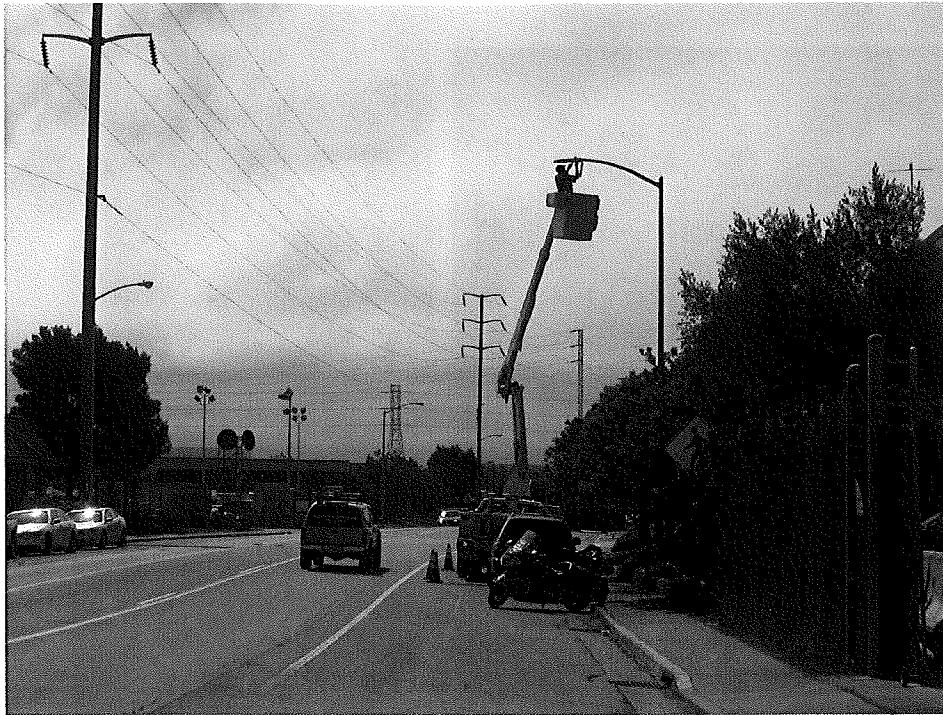
Replacing HPS Street Lights on Andersen Drive
