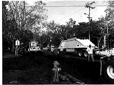
5 th Ave. During Construction
