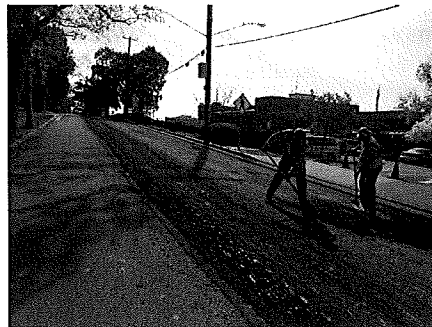
Mission Ave. Prep & Grinding
