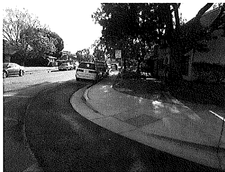
Kerner Completed Ramp
