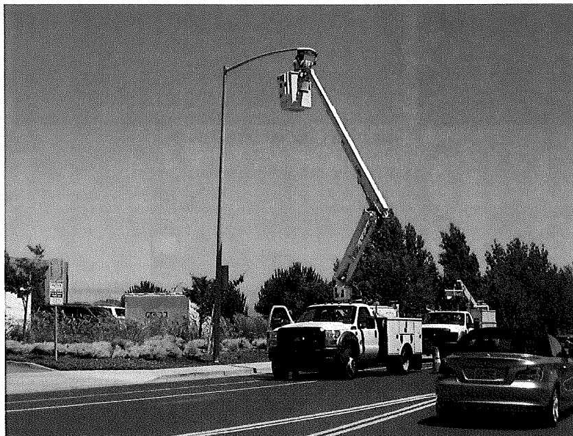
Replacing HPS Street Lighting on Kerner Blvd.
