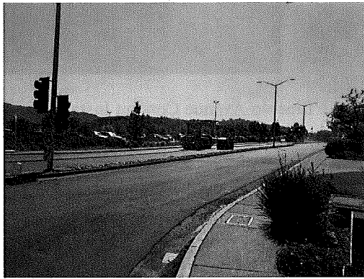
Roadway Paving – Northgate Drive
