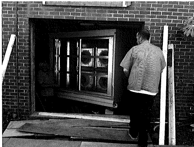
Cooling Roof Unit and Fan Installation
