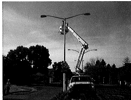
Installation of new Street Light - Canal
