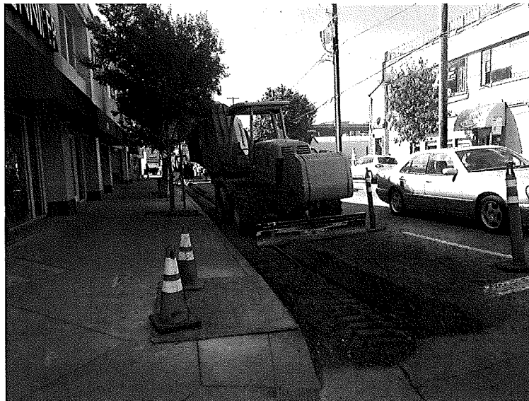
Lincoln Avenue Conduit Installation – Trenching prior to paving.
