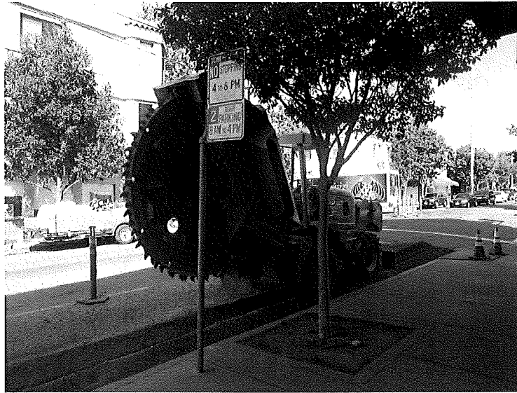
Lincoln Avenue Conduit Installation – Rock Wheel utilized to Cut Trench
