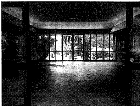
City Hall Entryway – During Construction
