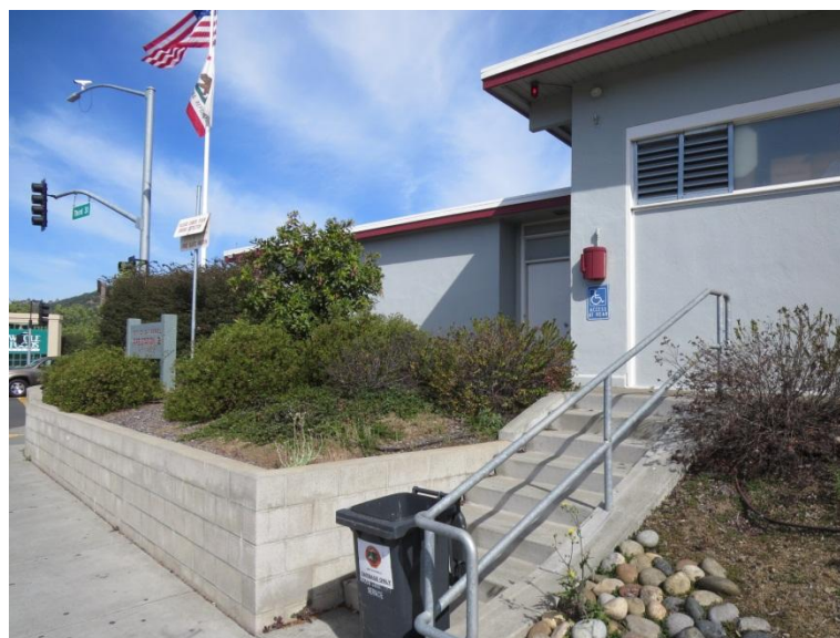
Photo 2: Station 52, Front View of the Entrance
