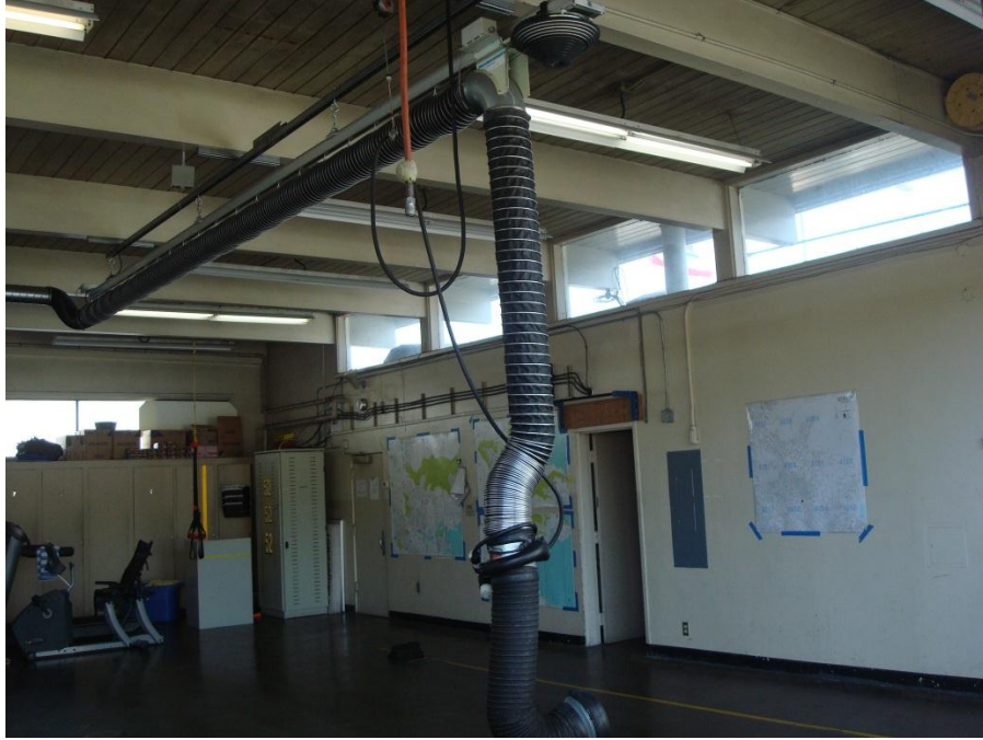
Figure E5: Communication Equipment Cabinet in Apparatus Bay
