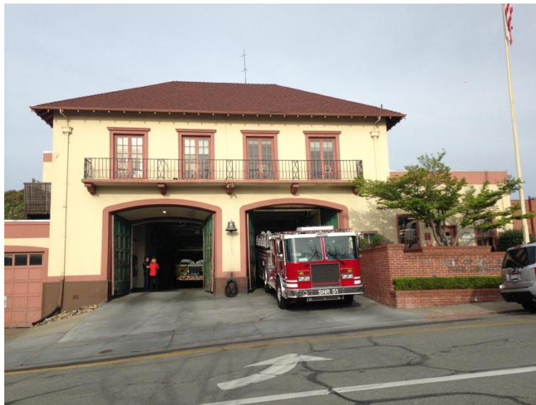
Photo 1: Station 51, Front View of Building
