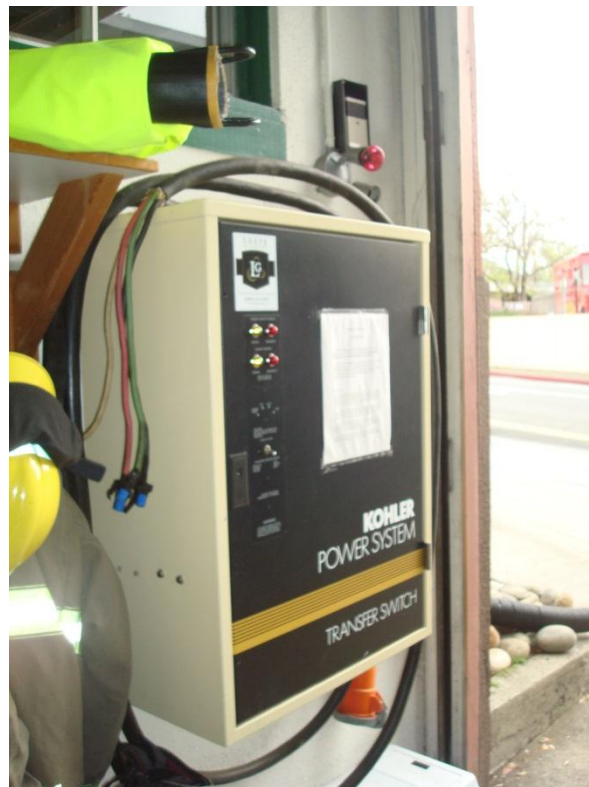
Figure E4: Automatic Transfer Switch with Cables for Portable Generator Connection
