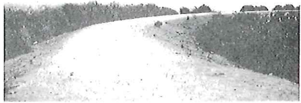
Photo 6: Typical Engineered Levee Along Spinnaker Marsh
