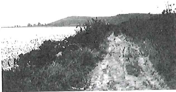
Photo 4: Existing Canalways Levee Top
