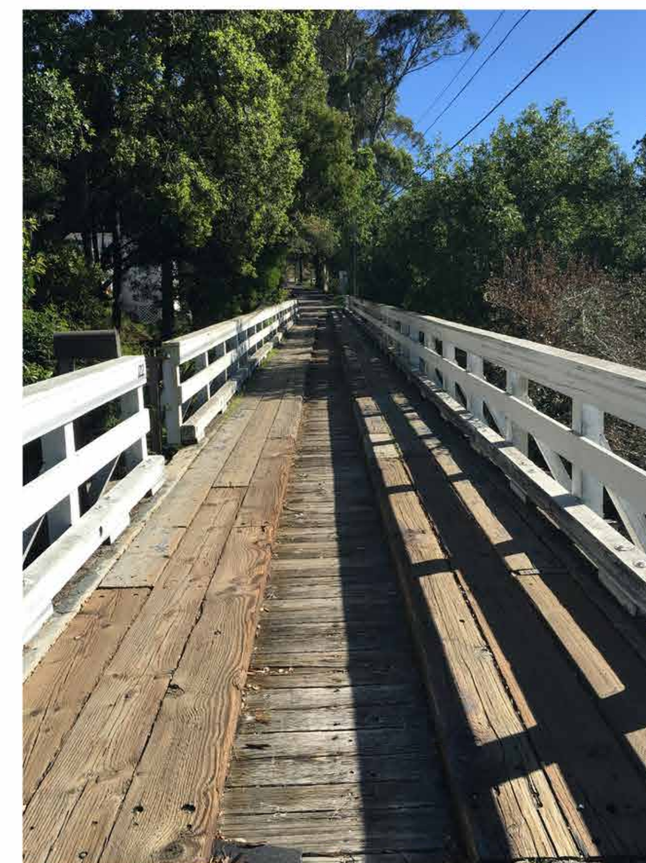
EXISTING BRIDGE SURFACE
