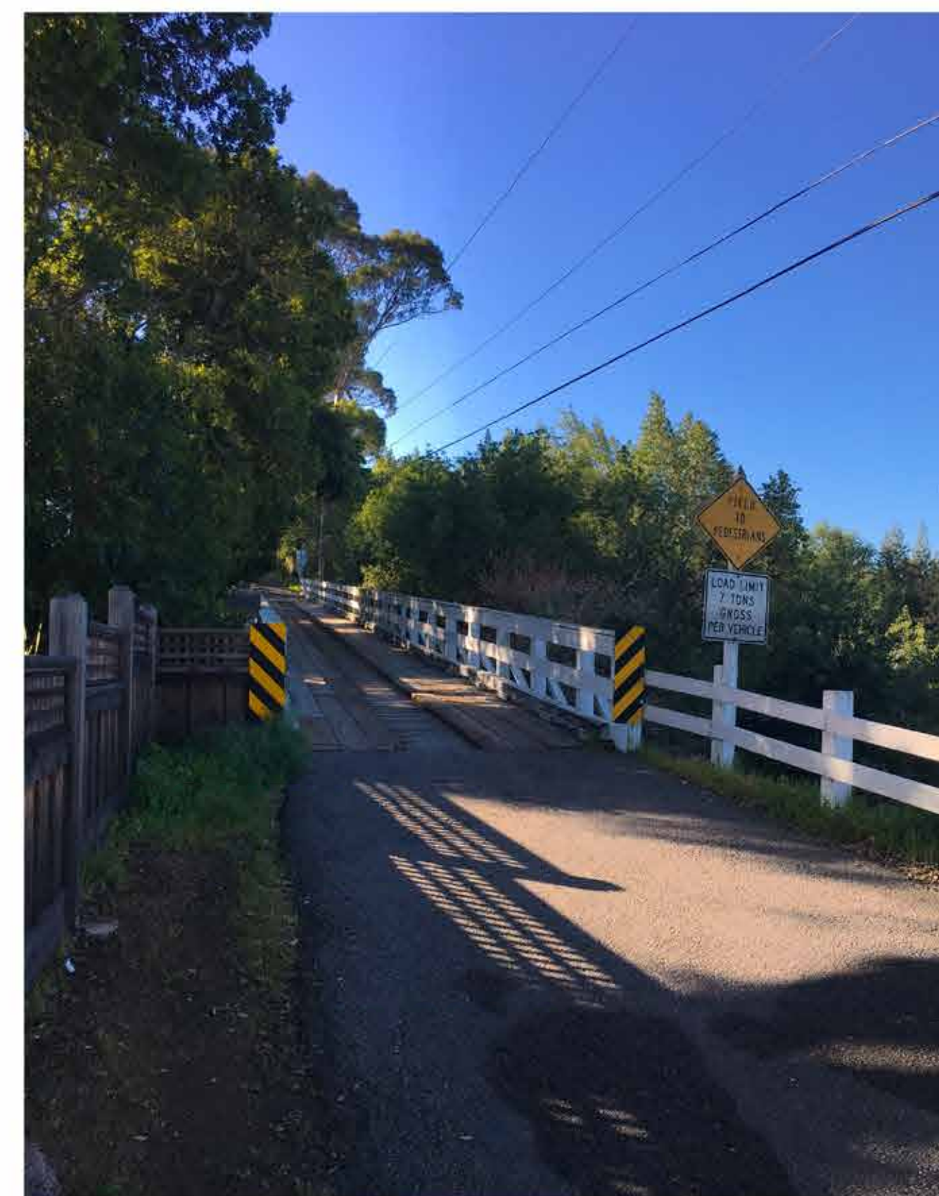
EXISTING NORTH END
