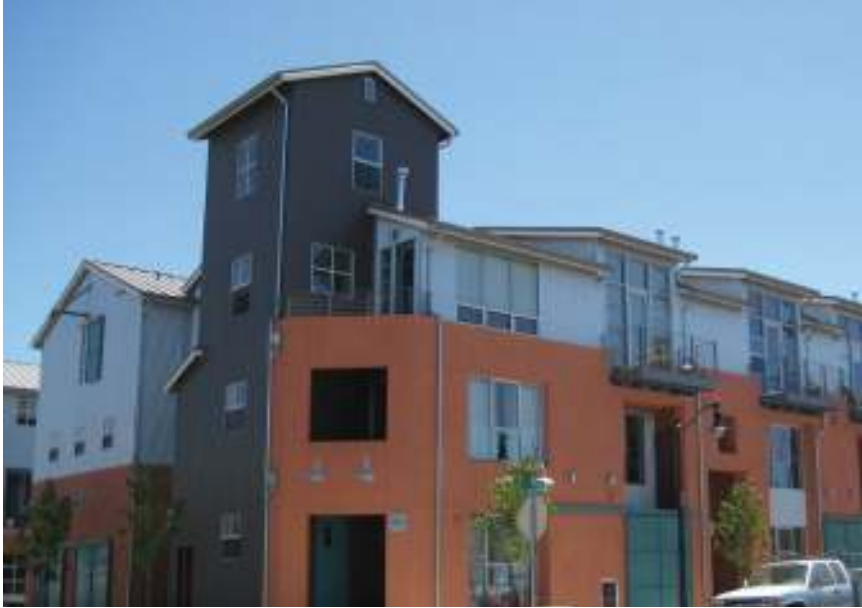
Variation in architectural materials and massing
