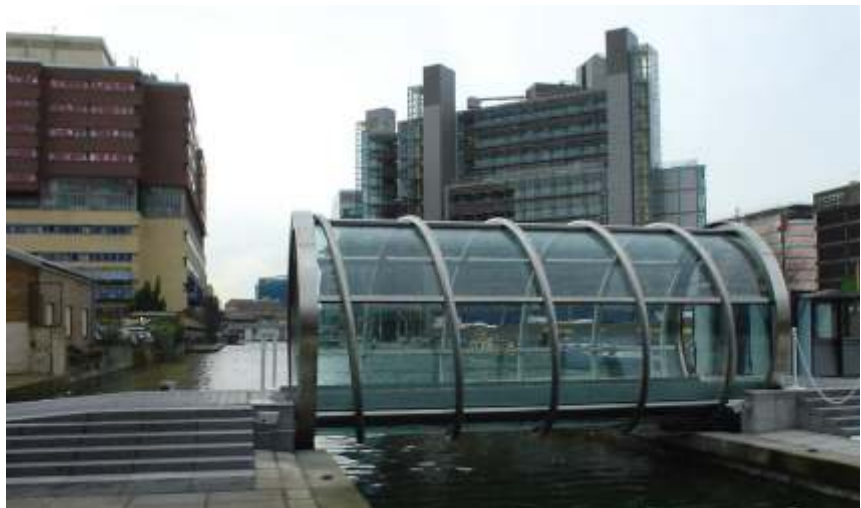
Example of an operable crossing
