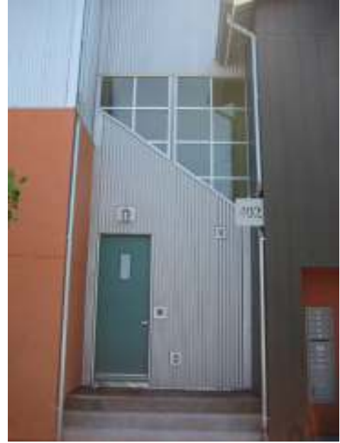
Building materials and color
