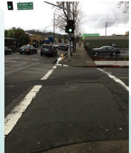
Figure 54: Standing water at curb ramp
