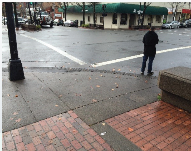
Figure 53: ADA non-compliant curb ramp
