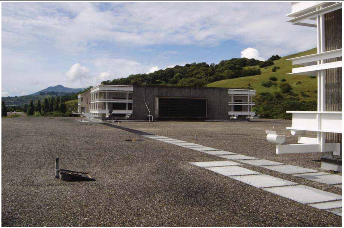
View of the roof and penthouse of the 1600 Los Gamos Drive building.
