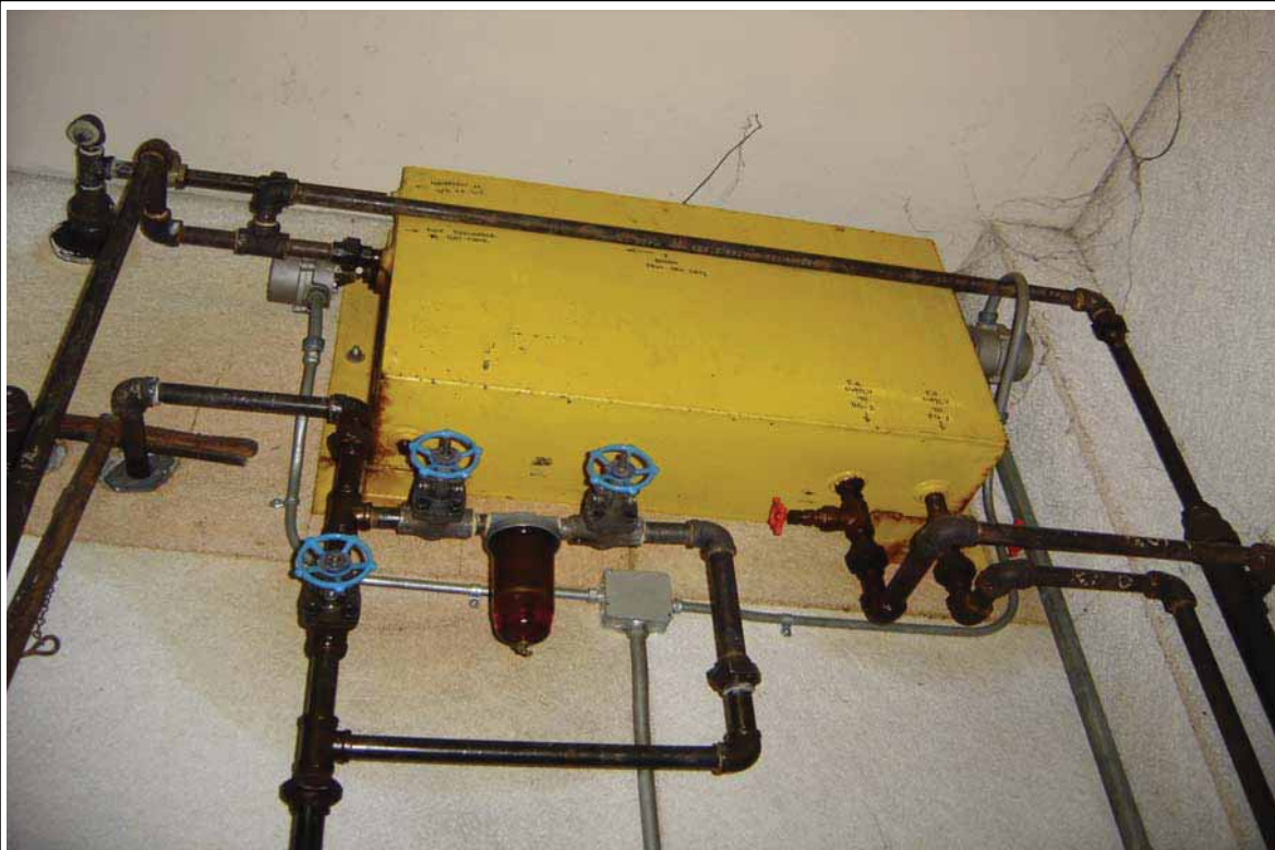
View of the day tank (wall mount) associated with the emergency backup generators.
