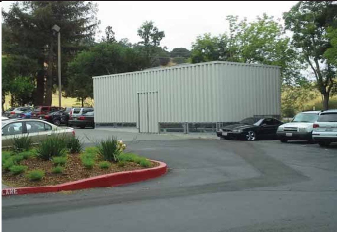
View of the Cooling Towers, located in the east parking lot.
