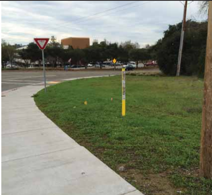
View of the gas pipeline warning sign located on the West Parcel.
