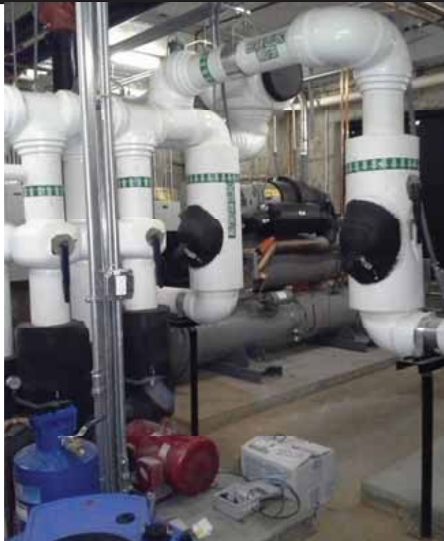
View of the Chiller Room.
