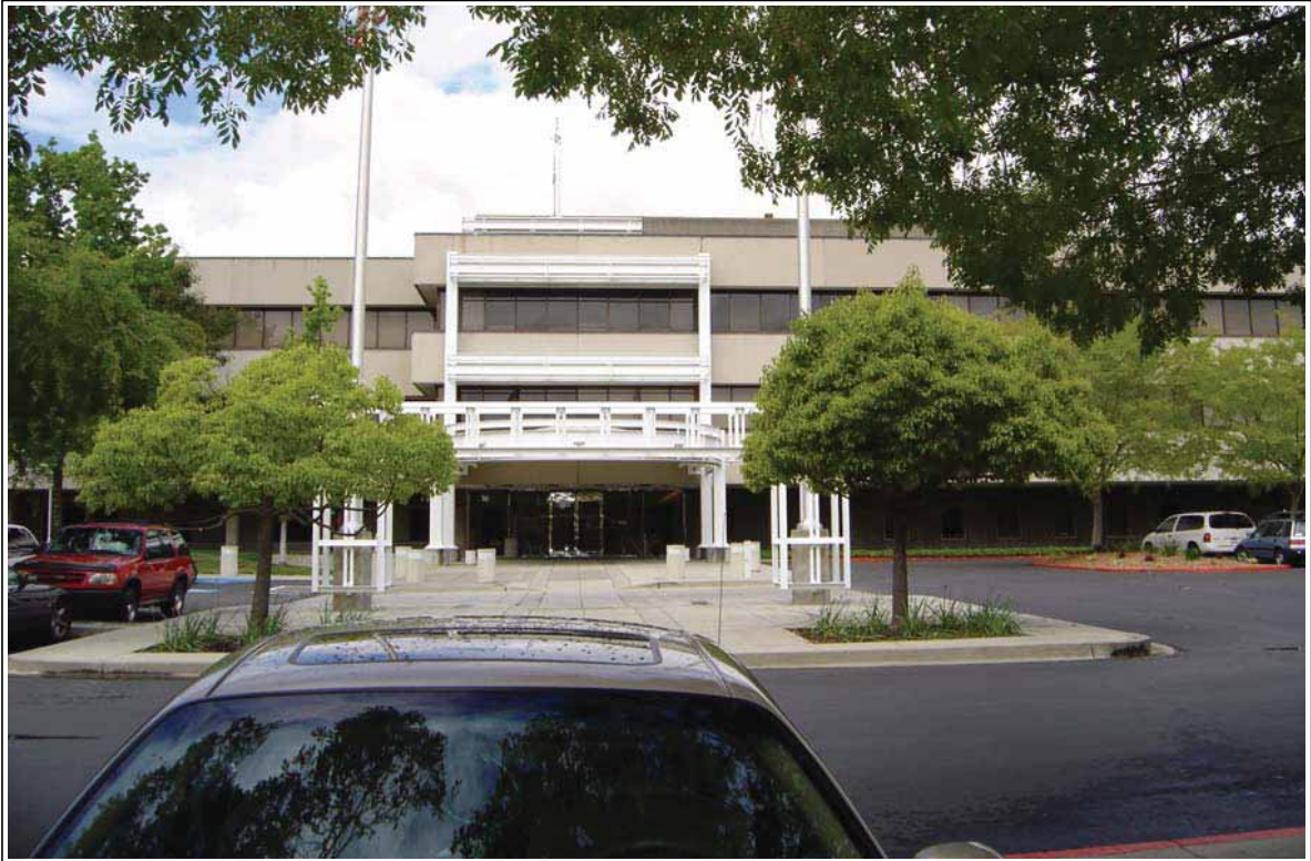
View west of the Lobby A entrance to the 1600 Los Gamos Drive building.
