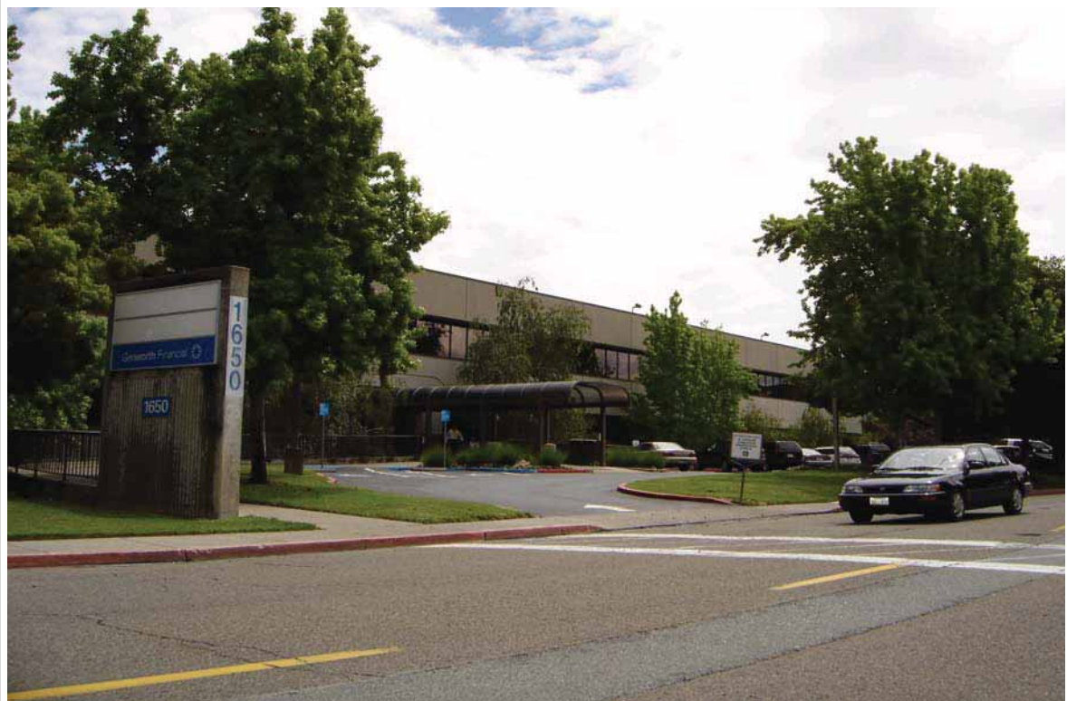
View southeast of the main entrance to the 1650 Los Gamos Drive building.
