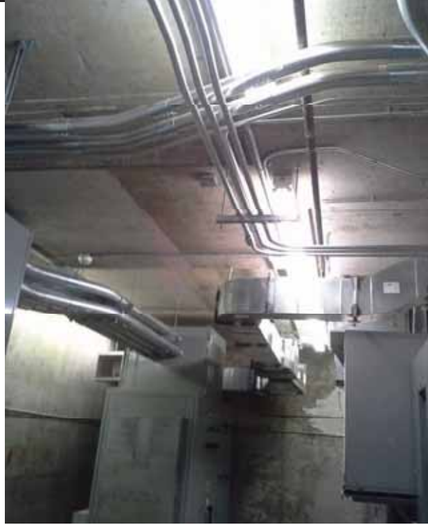
View of the Boiler Room.
