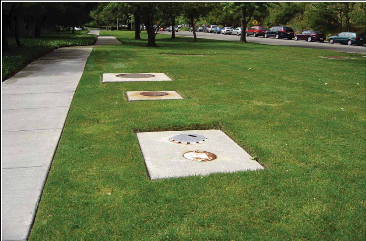
View of the UST location adjacent to the 1600 Los Gamos Drive building.
