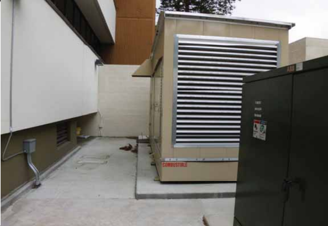
View of the generator and associated diesel AST, located at the southwest corner of the Property.
