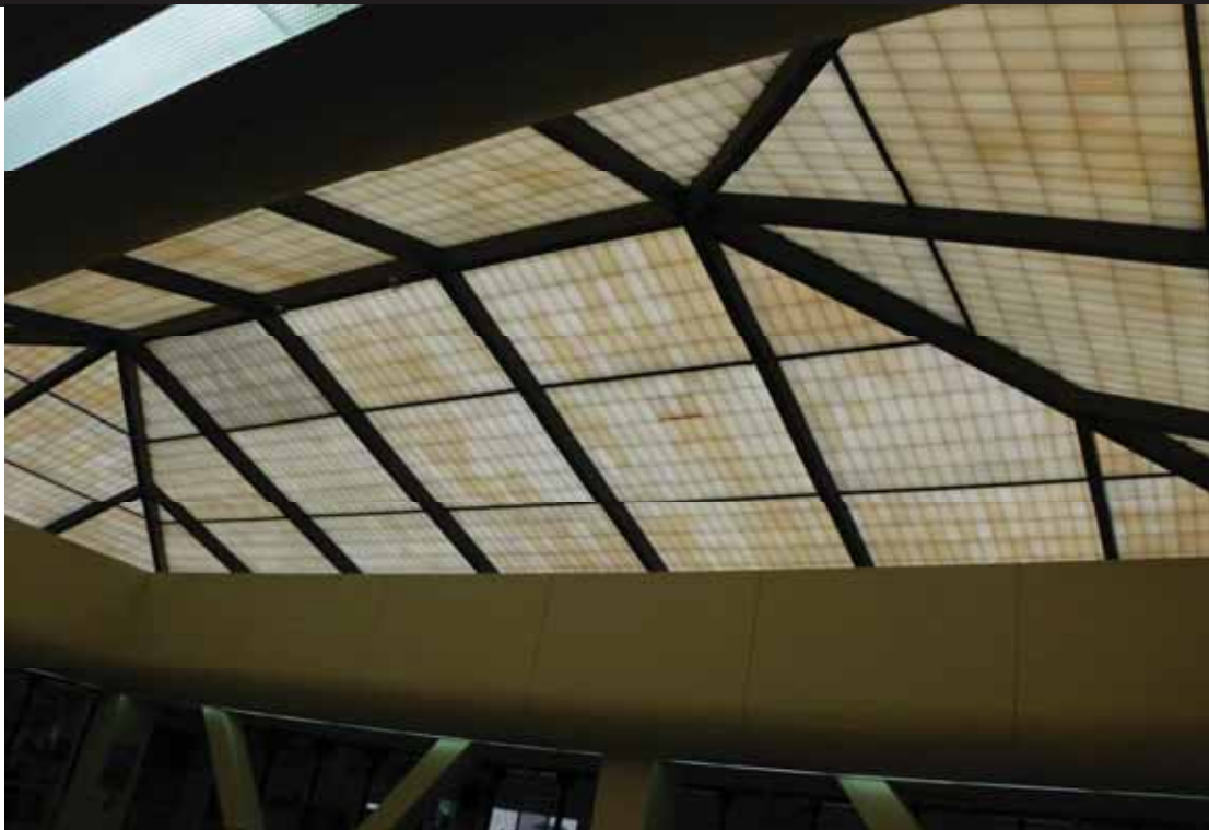
View of the building ceiling from Floor 3.
