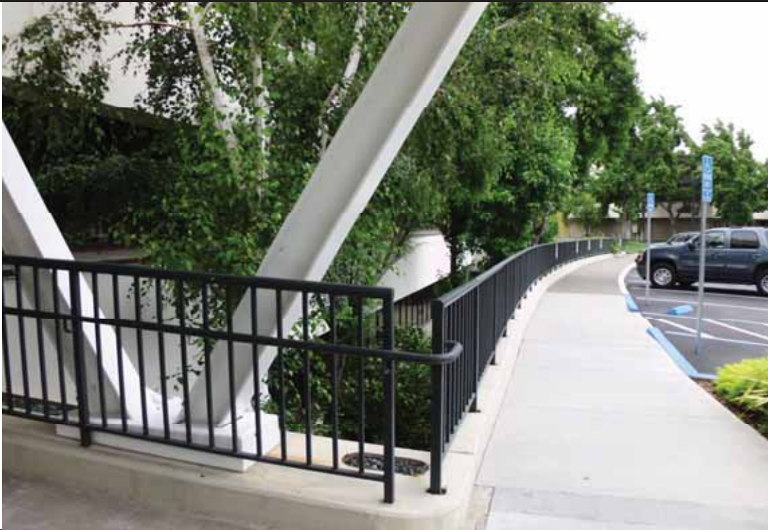
View of the entrance of the Property looking southeast.
