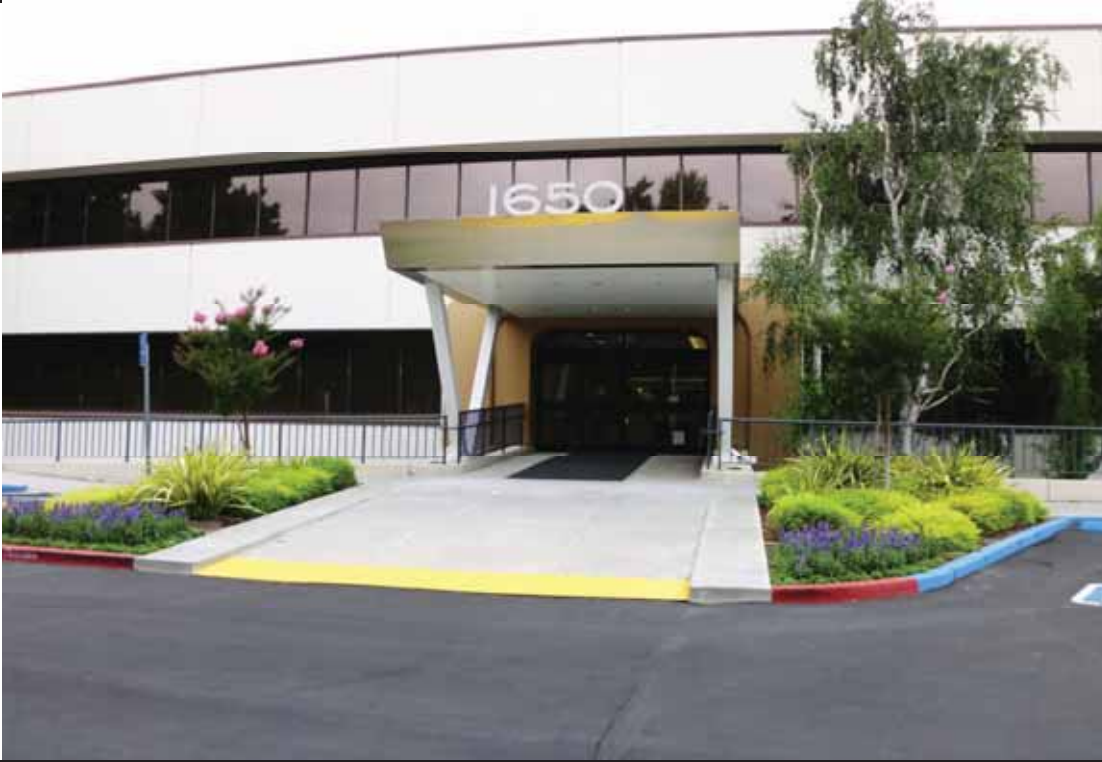
View of the entrance of the 1650 Los Gamos Drive building.
