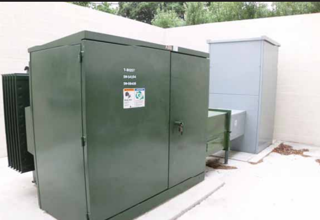
View of the transformer located in the southwest corner of the Property.
