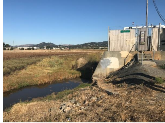
Figure 5 Drainage ditch from Hwy 101 feeding to pump station
