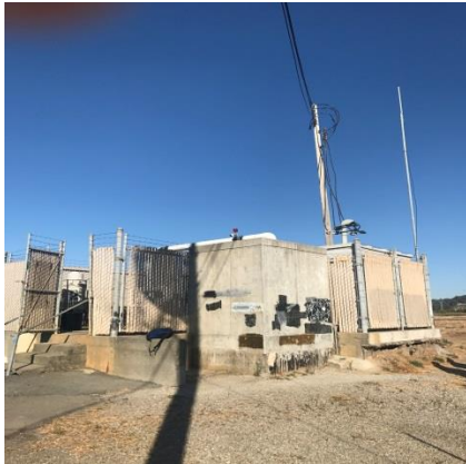
Figure 3 Pump Station is to be relocated then demolished
