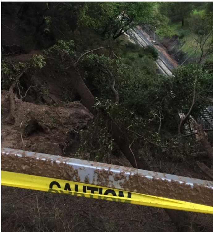
Figure 4-11 Area below Ranchitos Road looking toward the SMART Tracks
