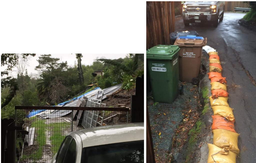
Figure 4-15 City of San Rafael Landslide near 201 Prospect and Southern Heights
