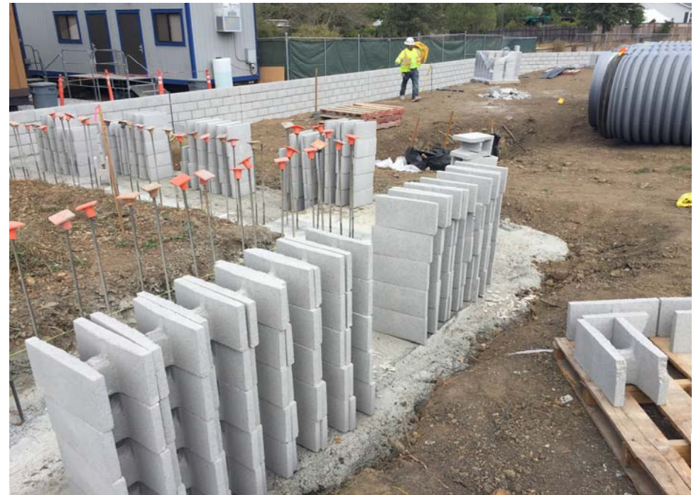
September progress pictures for Fire Station 57 – Retaining Wall construction
