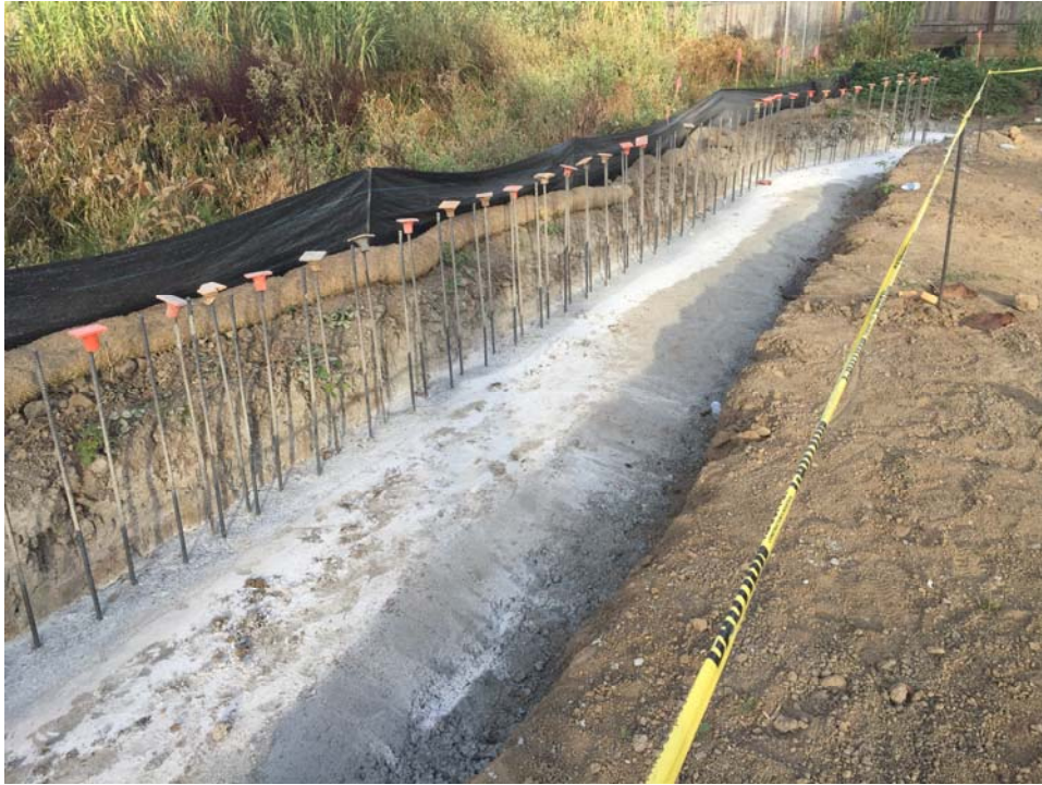
September progress pictures for Fire Station 57 – Retaining Wall Foundation
